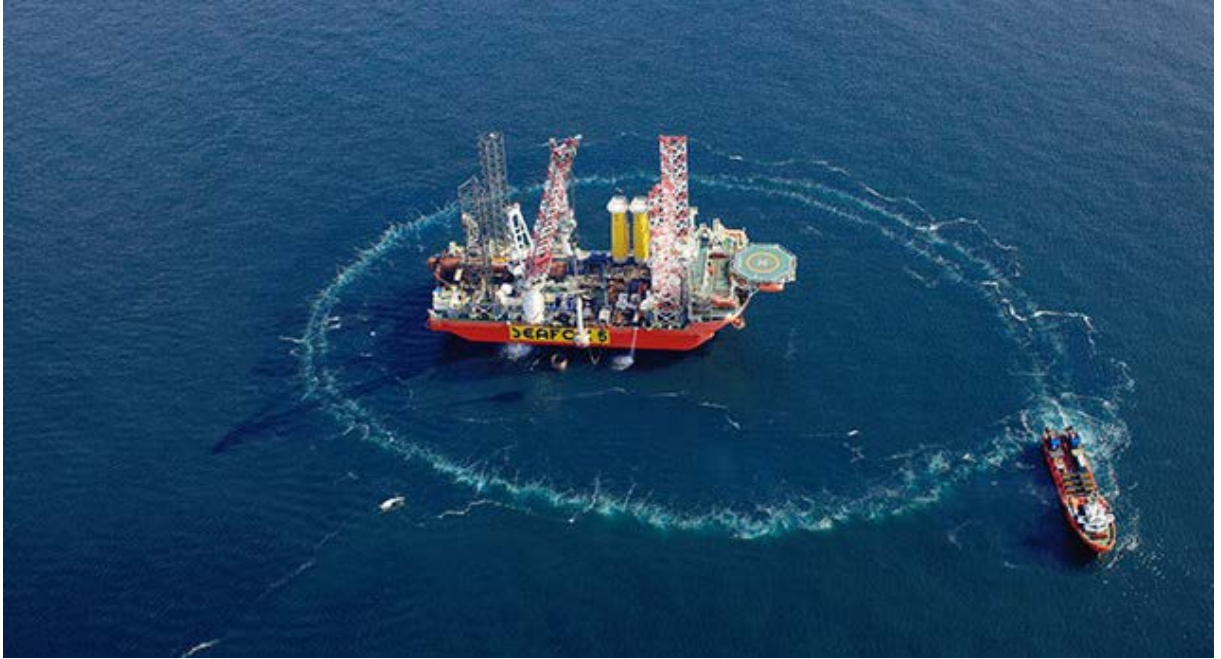
Figure 11.6: Bubble screen during the installation of offshore foundations
