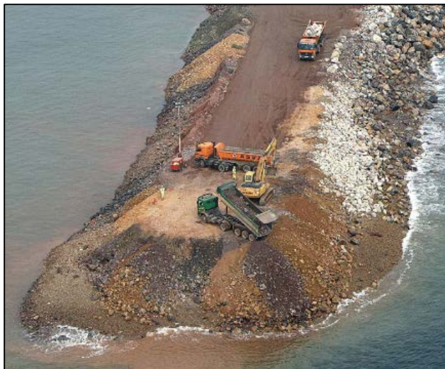
Figure 6 – Example of direct placement approach carried out by Dragados
