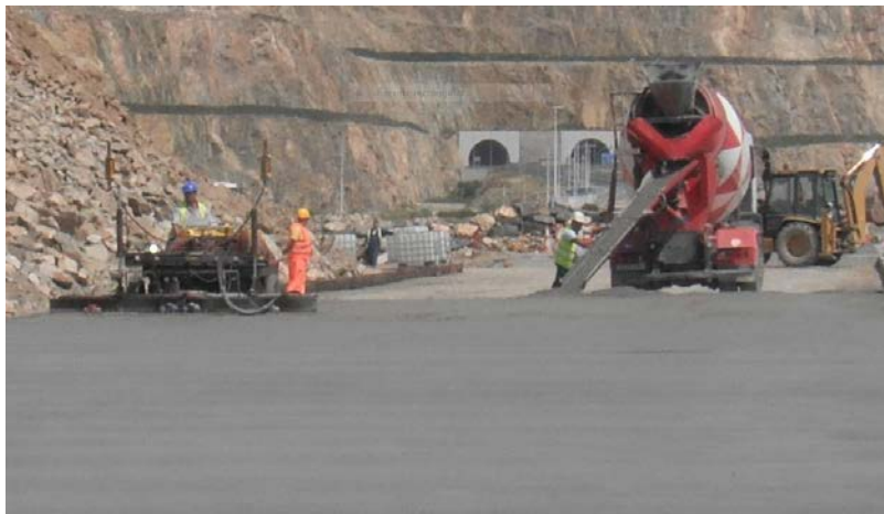
Figure 26 – Pavement construction activities
