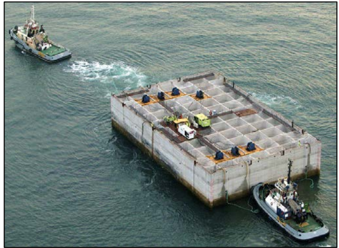
Figure 19 – Towage of Caissons to site
