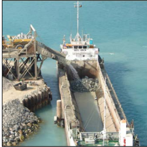
Figure 7 – Example of quarry vehicles loading a split barge hopper for future discharge
