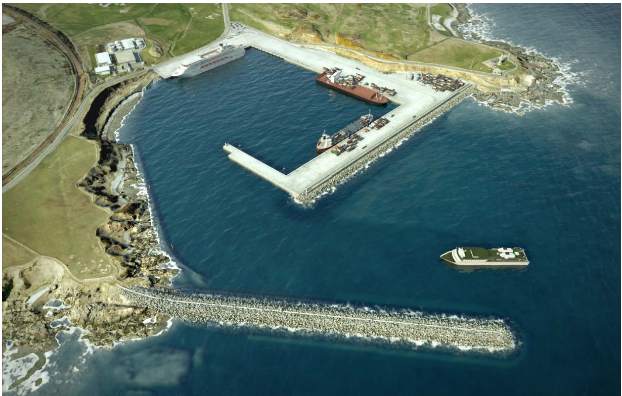
Figure 2 – Imposed aerial view of the bay after completion of construction
