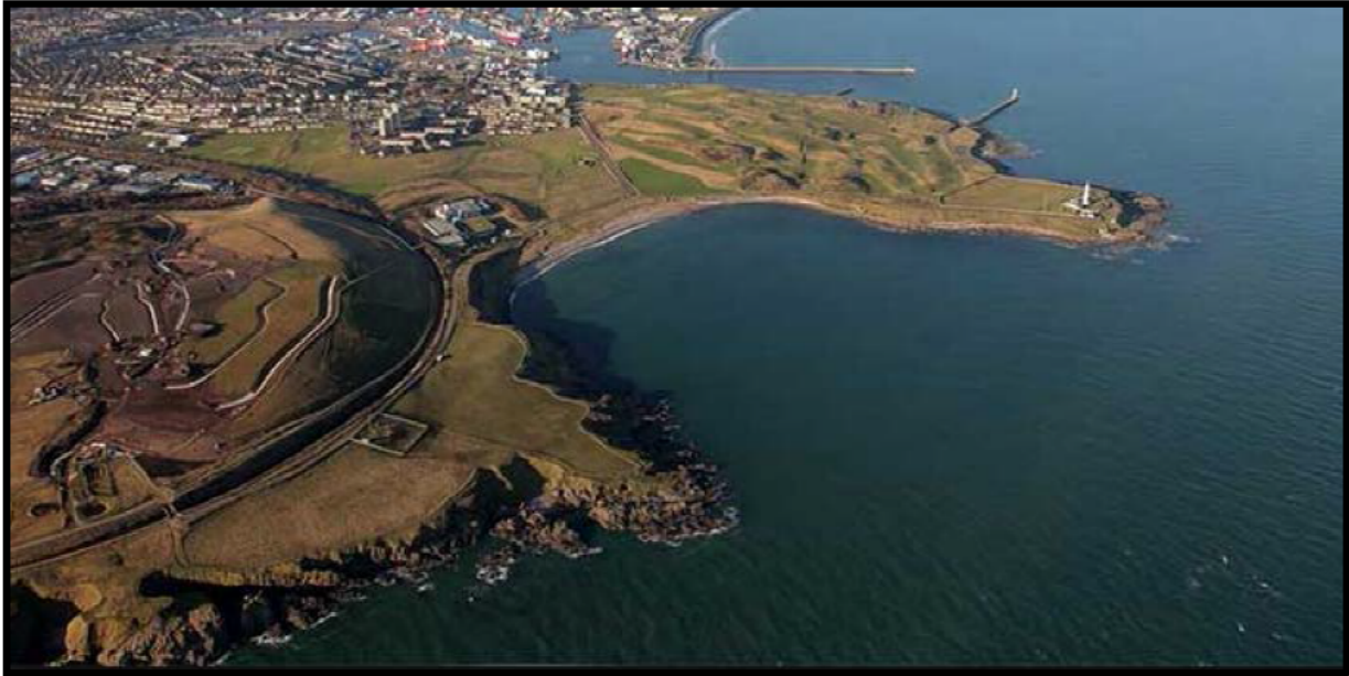
Figure 1 – Aerial view of the bay prior to construction
