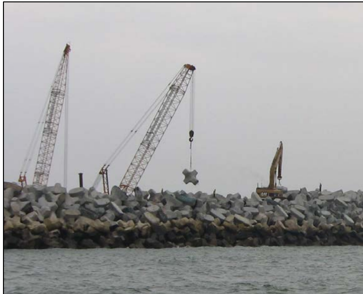
Figure 9 – Placement of Accropode units
