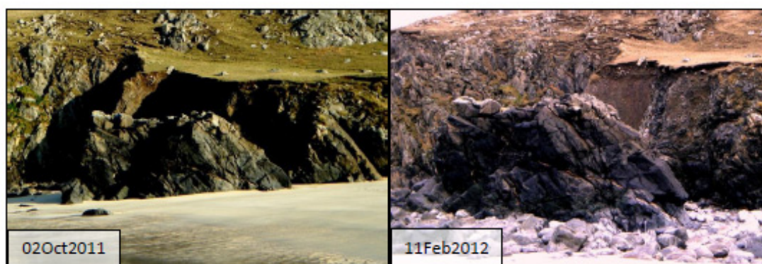
Plate 7.1 Observed beach changes at Dalmore Oct 2011 and Feb 2012
