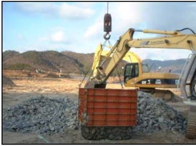
③ Lift up the production frame and leave Filter Unit. Production is finished.
