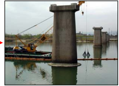
⑤ Installation by a crane.
