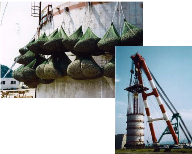
Example of work: Protection of bridge foot
