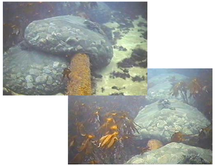
Example of work: Pipeline protection
