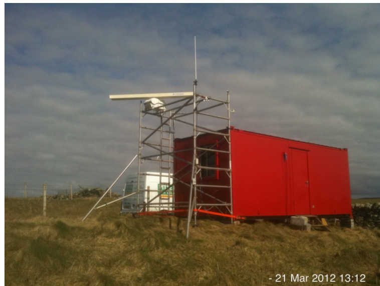
Figure 17 Radar/AIS Survey Station
