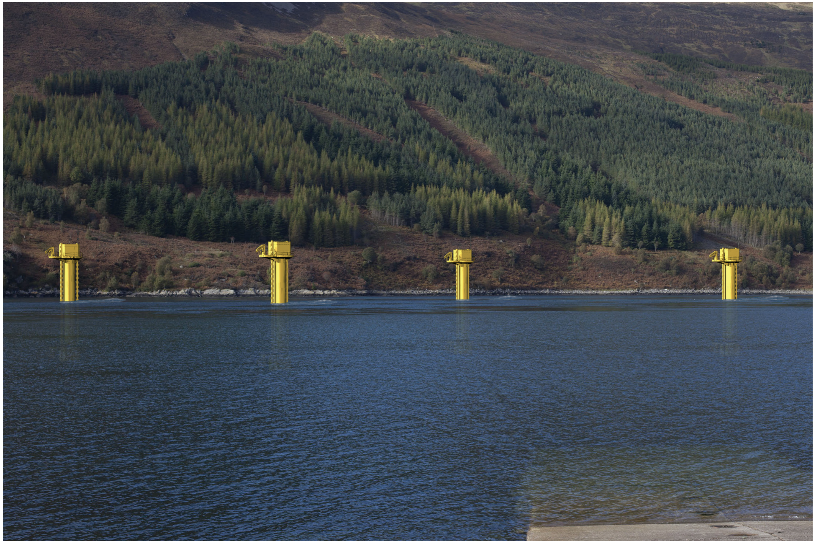
Fig 16.4.2g - VIEWPOINT 2 FERRY CROSSING EAST
