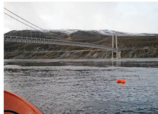
Figure 7 Measuring from a fixed mooring position close to land (south). The Kvalsund Bridge is in the background. The tidal turbine is about 200 m behind the floating buoys. The floating buoys are attached to the mooring and to the boat. The picture is taken during strong currents towards east (rising tide) 22 nd October 2009. The measuring boat is located in calm water, by the compensation current, and is right here drifting towards land.
