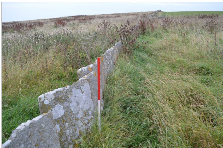
Plate 2: Traditional Caithness flagstone dyke (ORCA No. 58), looking east
