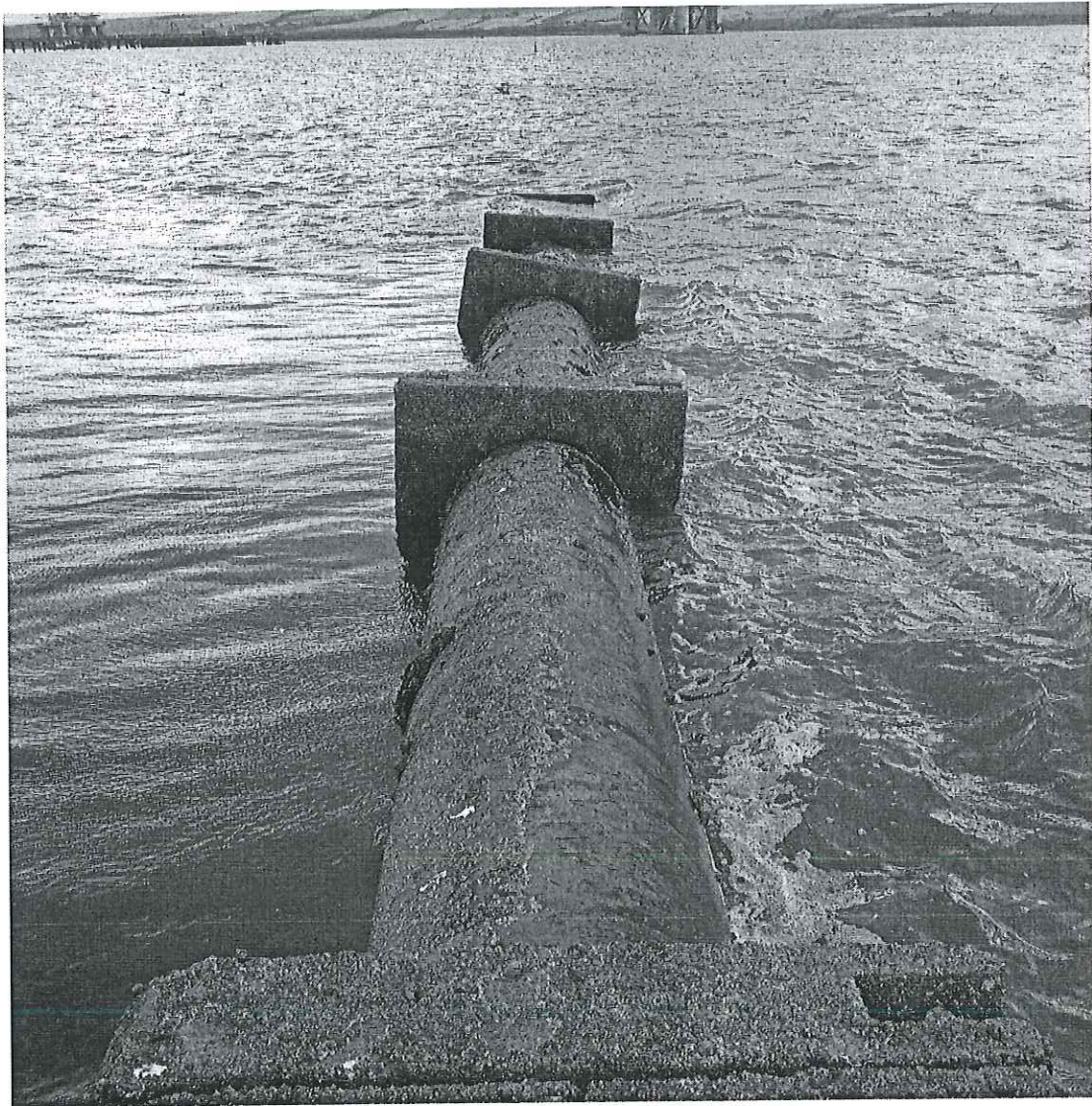
Photo 1 - View looking south along the existing outfall, end marker visible in the distance. Image taken at mid-tide.
