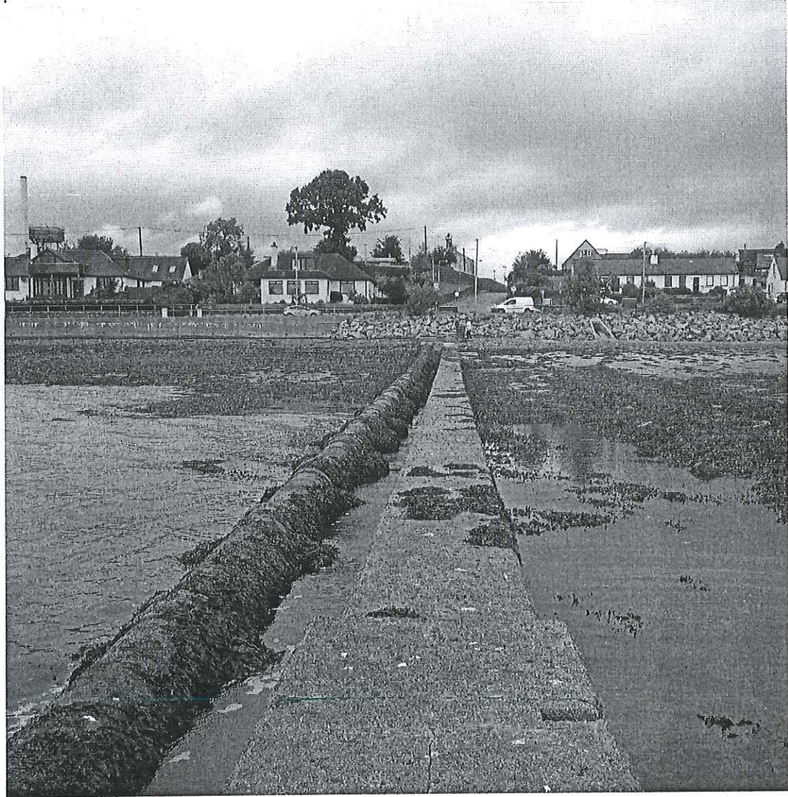
Photo 2 – View looking north along the existing outfall, personnel at shore chamber.
