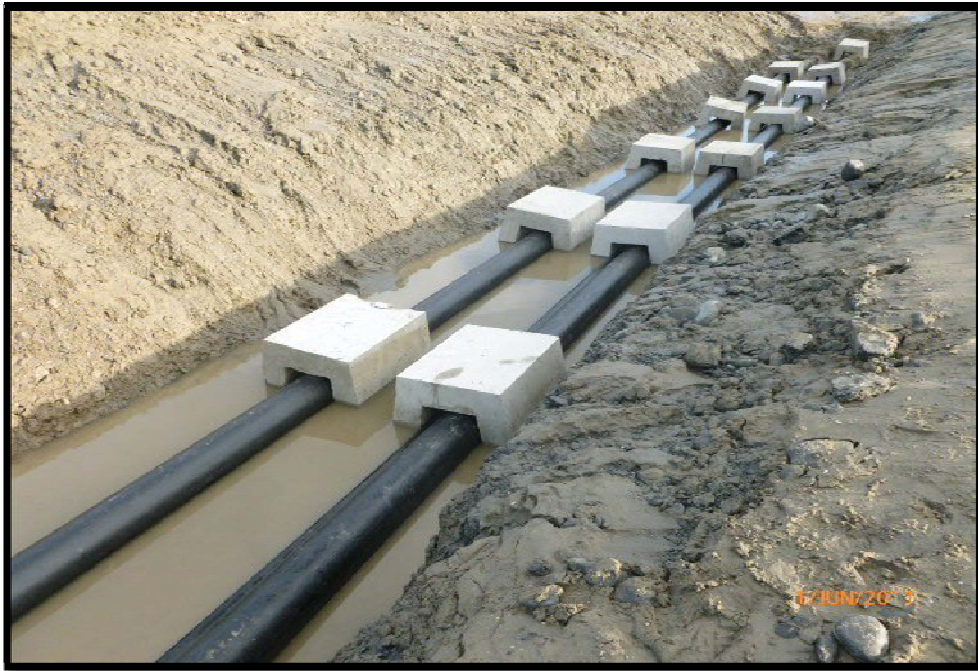
Figure 4: Open Cut Trench Cable Installation
