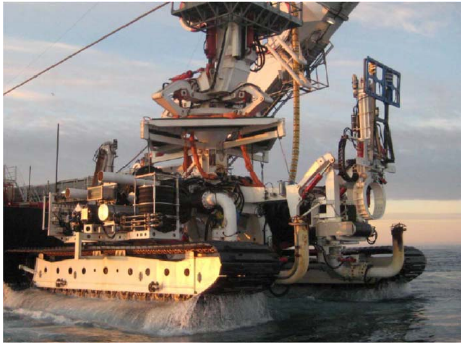
Figure 5-25: Typical cutting and jetting tracked burial tool
