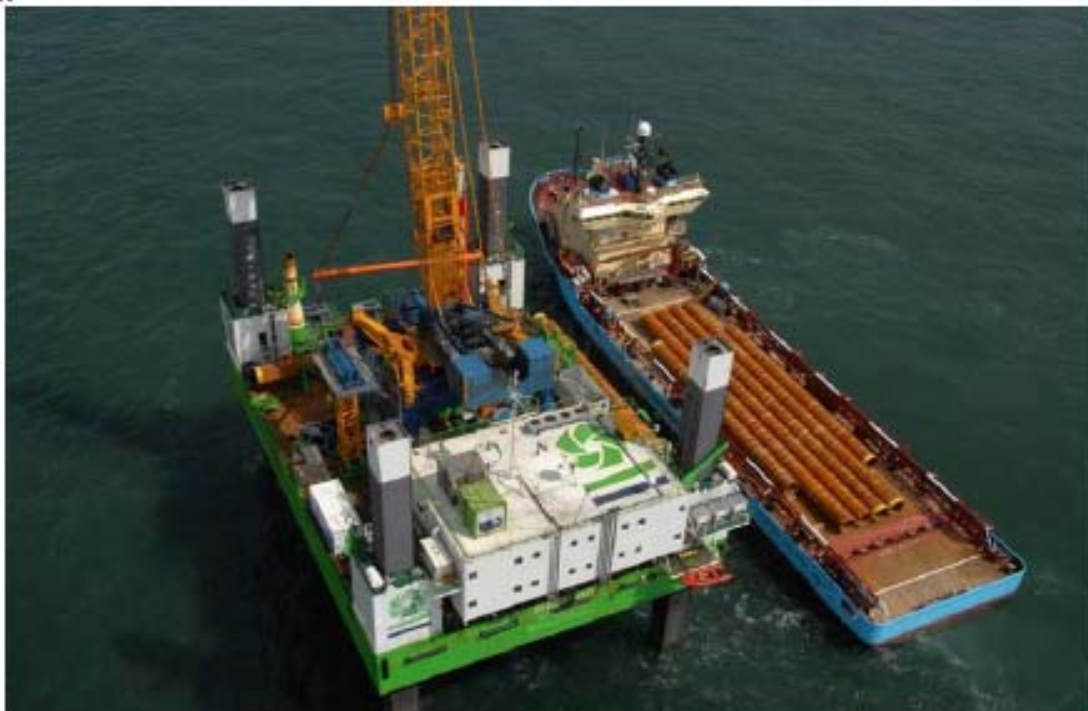
Figure 5-8: PSV Pile Delivery
