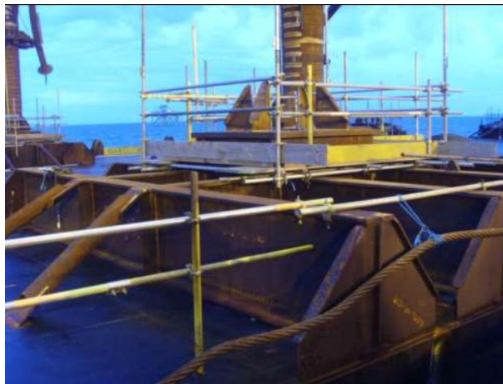
Figure 5-14: Sea fastening of Jacket
