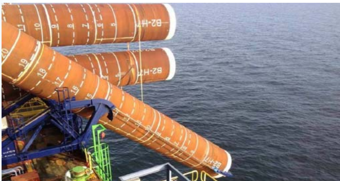
Figure 5-9: Saddle & Hook System for upending piles
