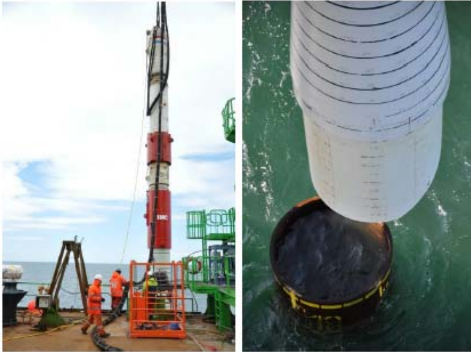
Figure 5-11: Pile Driving
