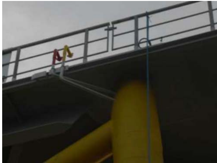
Figure 5-16: Connection point on jacket for grouting
