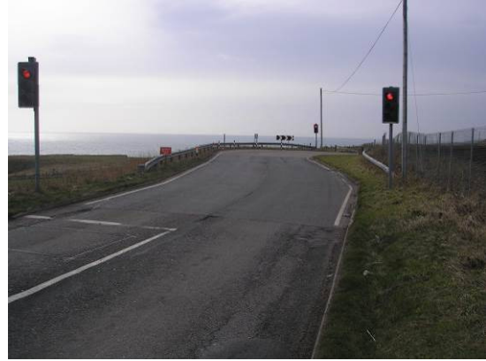
Coast Road Railway Bridge Southbound Approach
