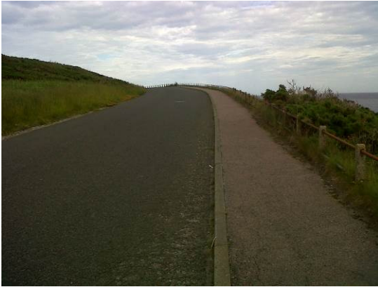
Footway on Greyhope Road Looking East 340m from Coast Road
