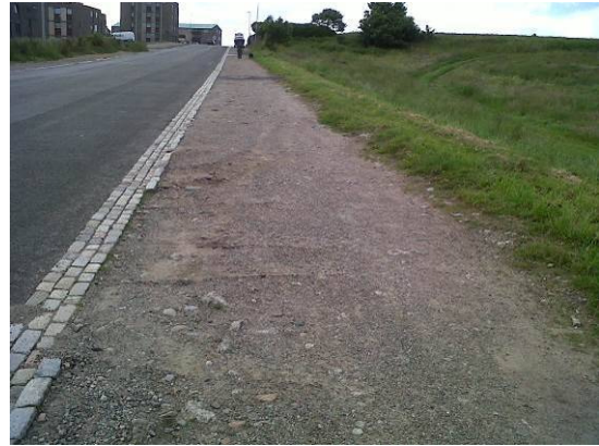
St Fittick’s Road Footway Construction
