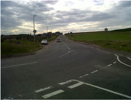
Footways on St Fittick’s Road Looking West from Greyhope Road
