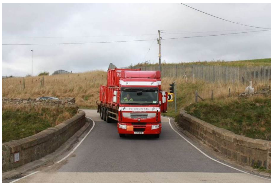
Coast Road Railway Bridge
