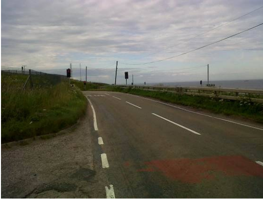
Coast Road Railway Bridge Northbound Approach
