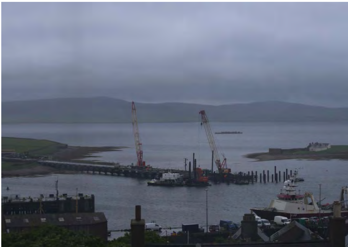
Figure 6.2 Stromness Harbour, Copland's Dock under construction
