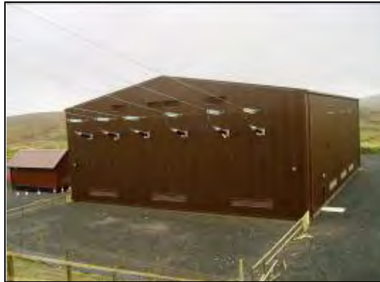
Figure 4.13 Example enclosed 132kV substation
