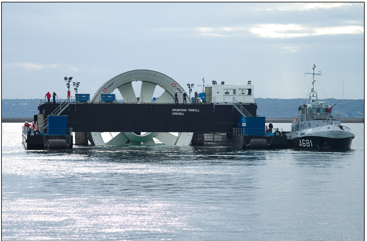
Figure 4.4 16m OCT being towed out to site in France
