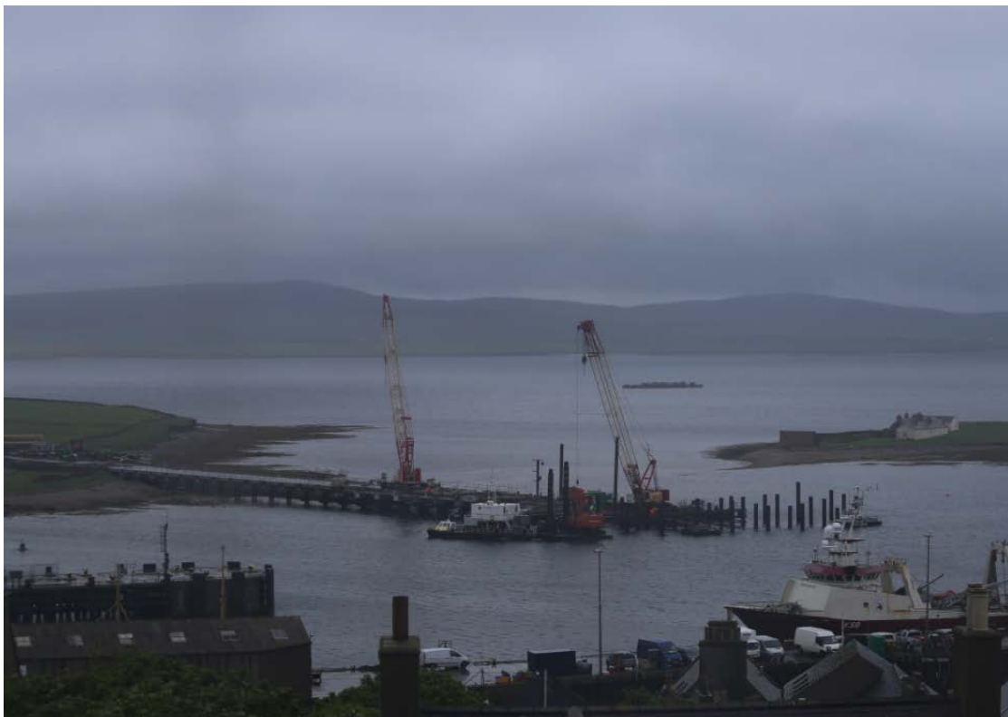
Figure 6.2 Stromness Harbour, Copland's Dock under construction
