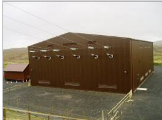
Figure 4.13 Example enclosed 132kV substation
