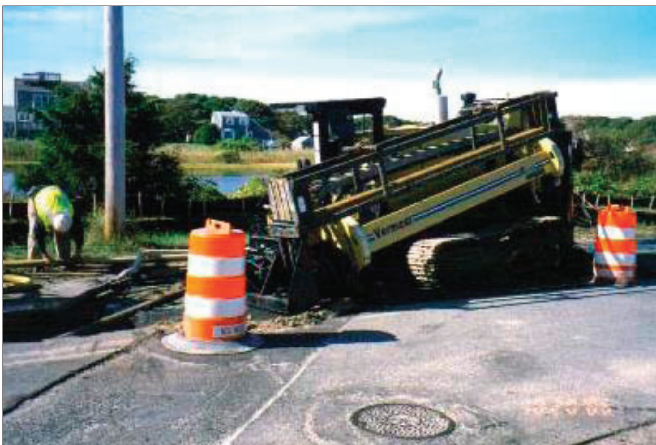
Typical HDD rig used for the installation of underground power cables
