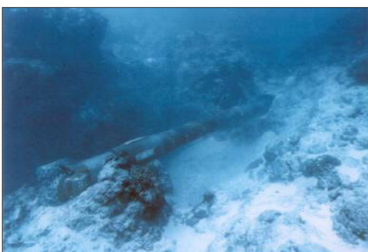
↑ Drilling head exit
