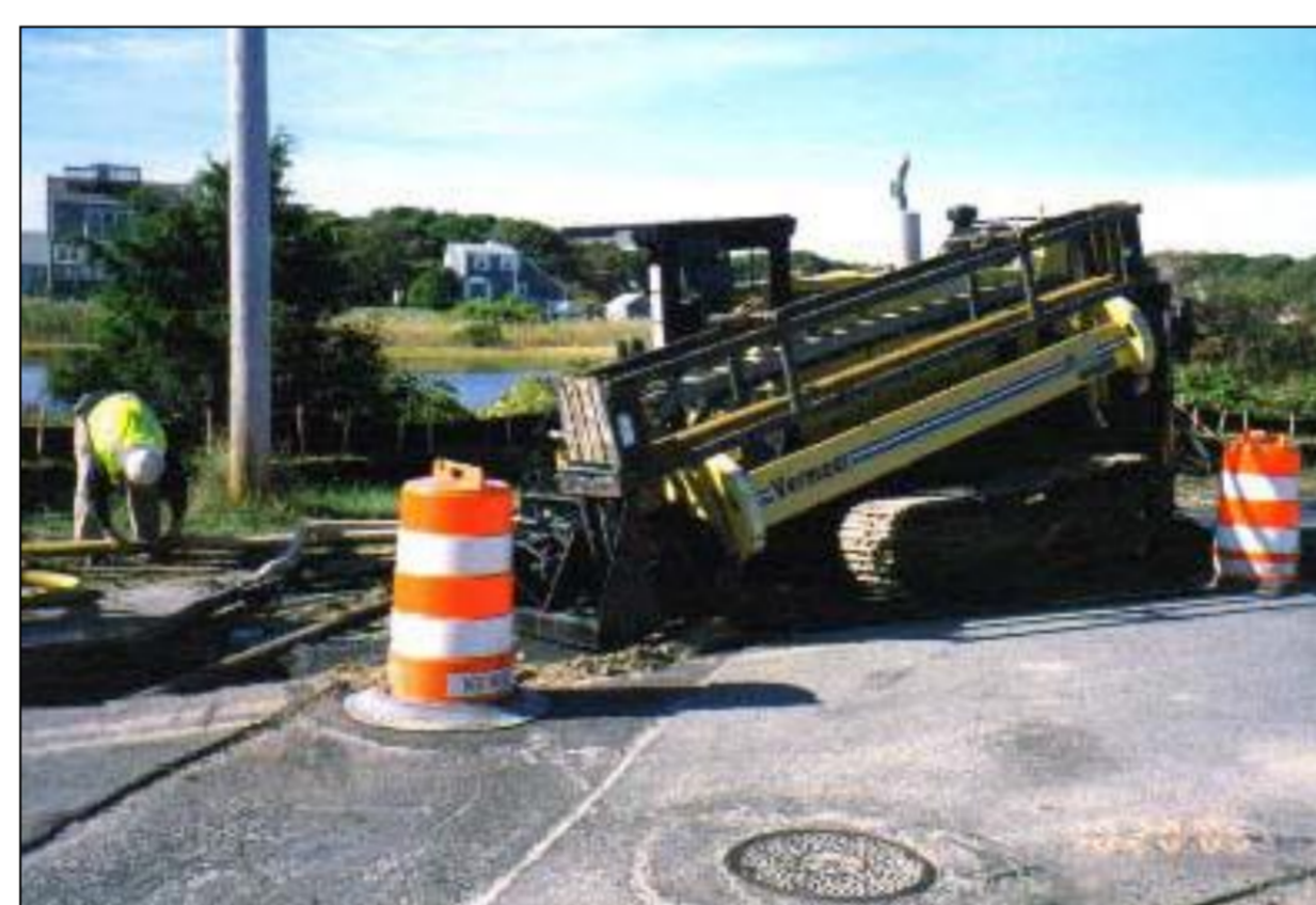
↑ Typical HDD rig for power cables
