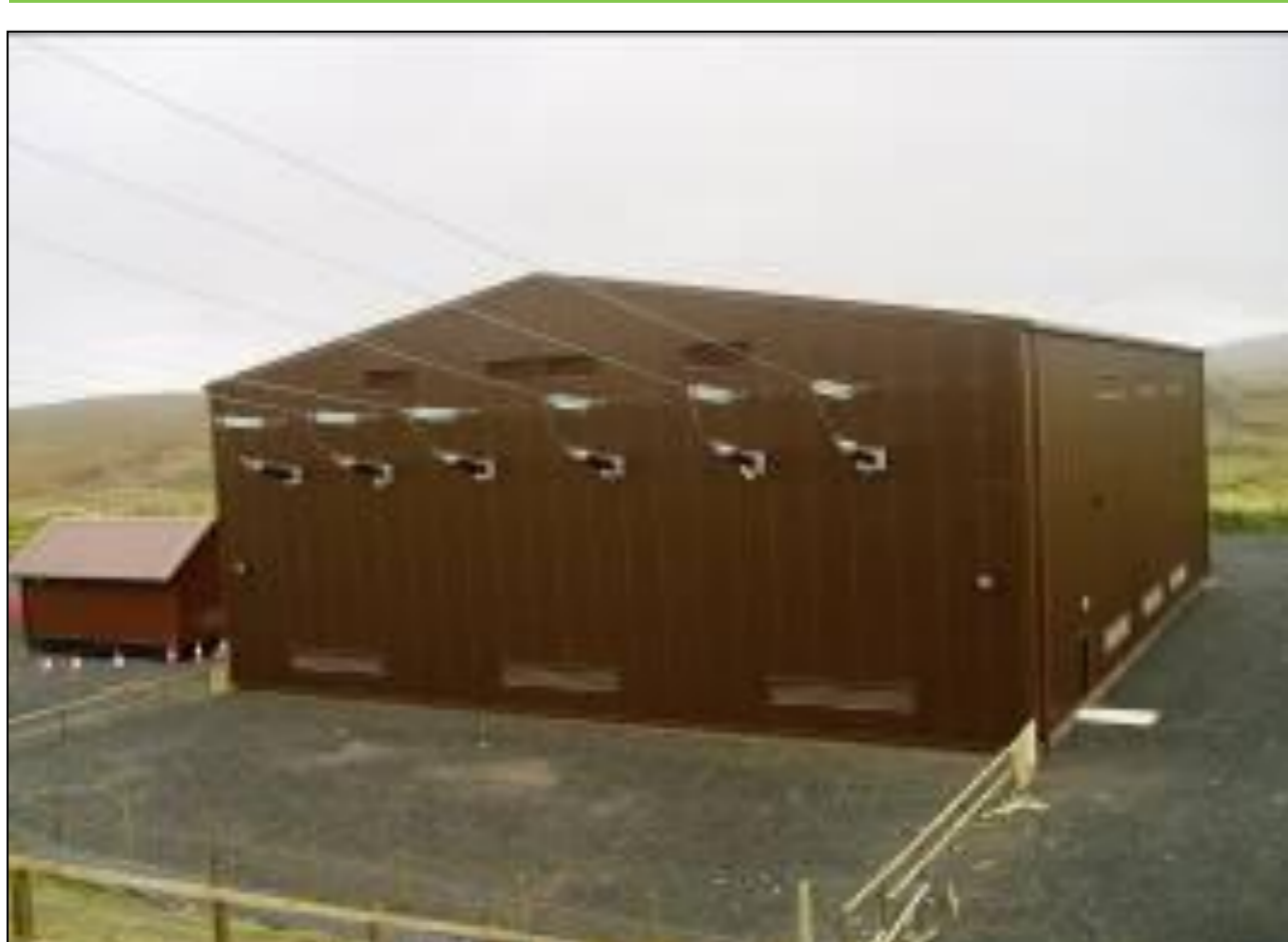
↑ Example of 132/33kV indoor substation building
