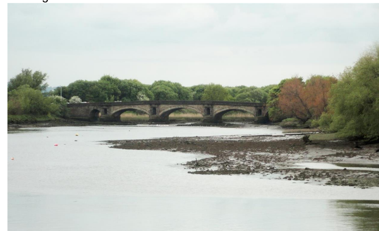
Photograph 15: The Listed Black Cart Bridge
