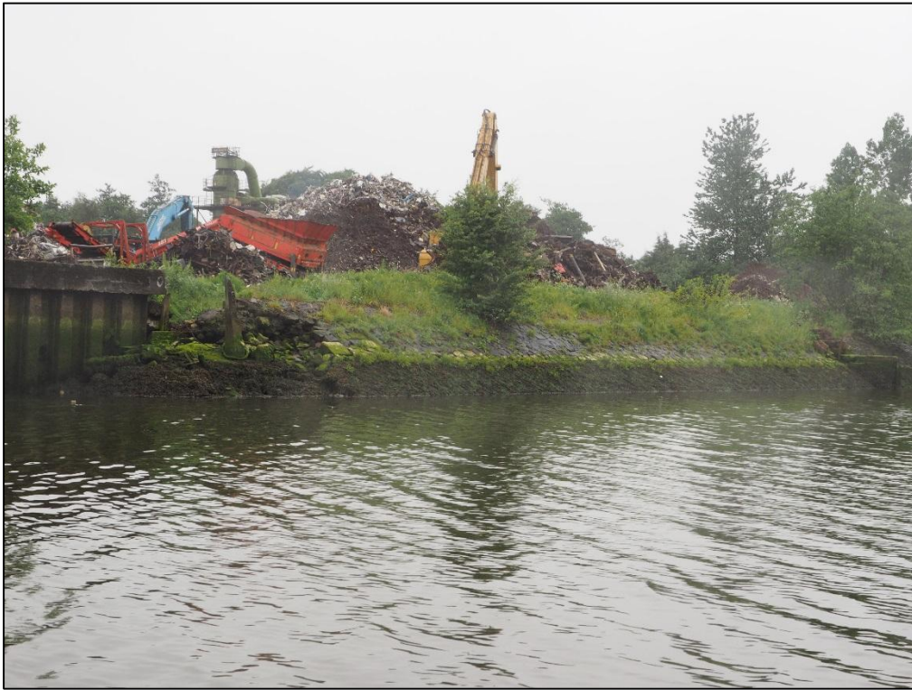
Photograph 3: Main Crossing South Pier Location East of Lobnitz Dock
