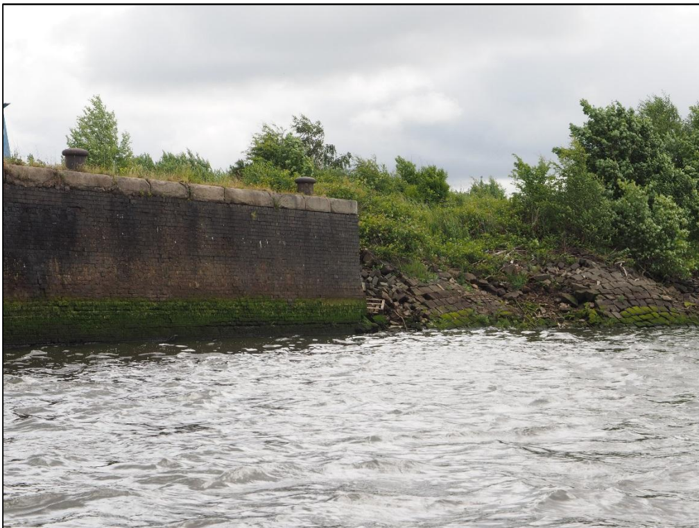
Photograph 4: Layby Berth Location Adjacent to Existing Rothesay Dock Quay Wall
