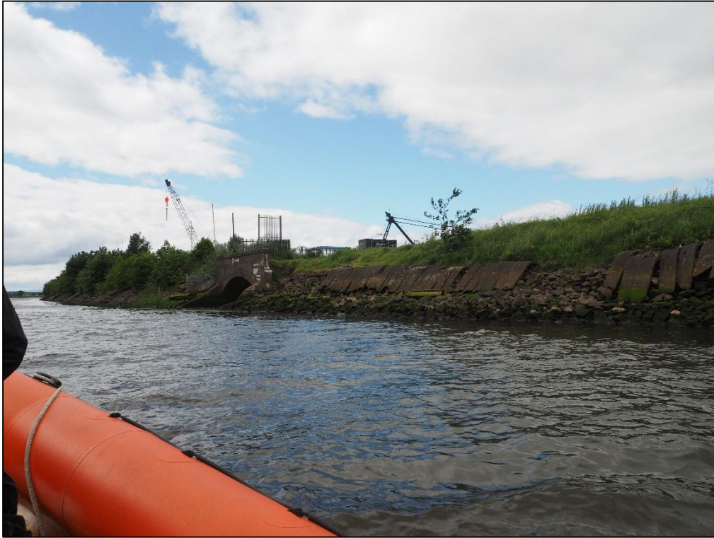
Photograph 1: Proposed Yoker Burn Culvert Realignment Outlet Position – East of Existing Culvert Outlet
