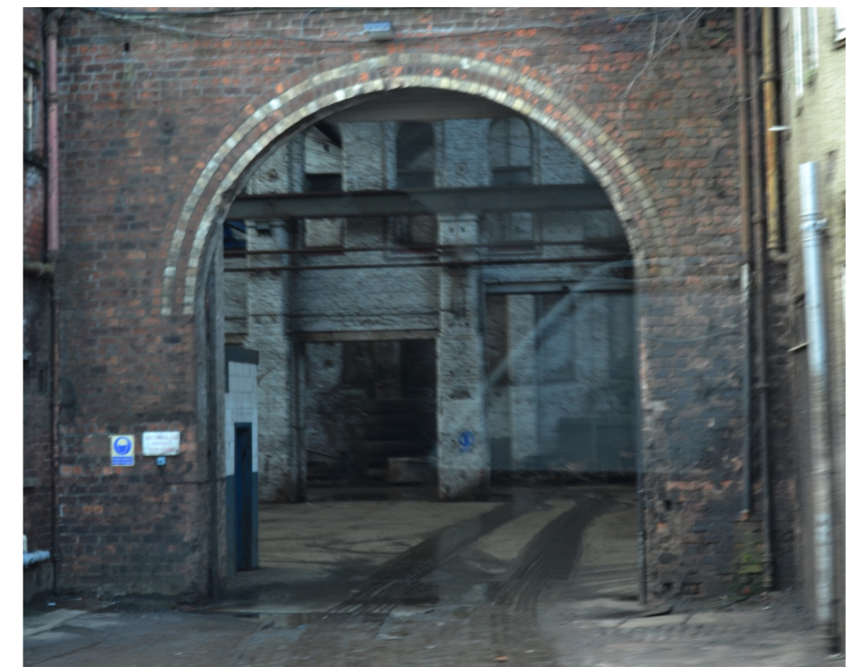
Arched entranceway into building
