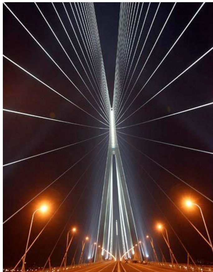
CLASH BETWEEN EXISTING AND FEATURE LIGHTING
