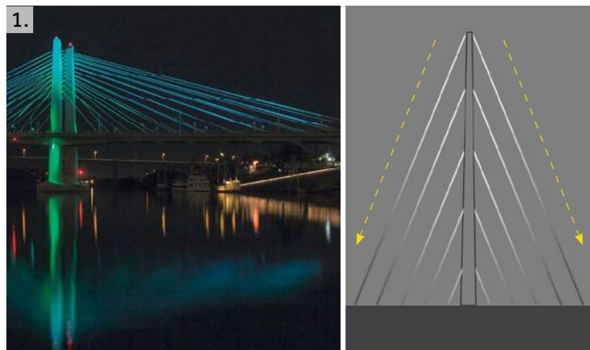
1. WASHING LIGHT DOWN Allows for a high level of control with no possibility of upwards light pollution.
