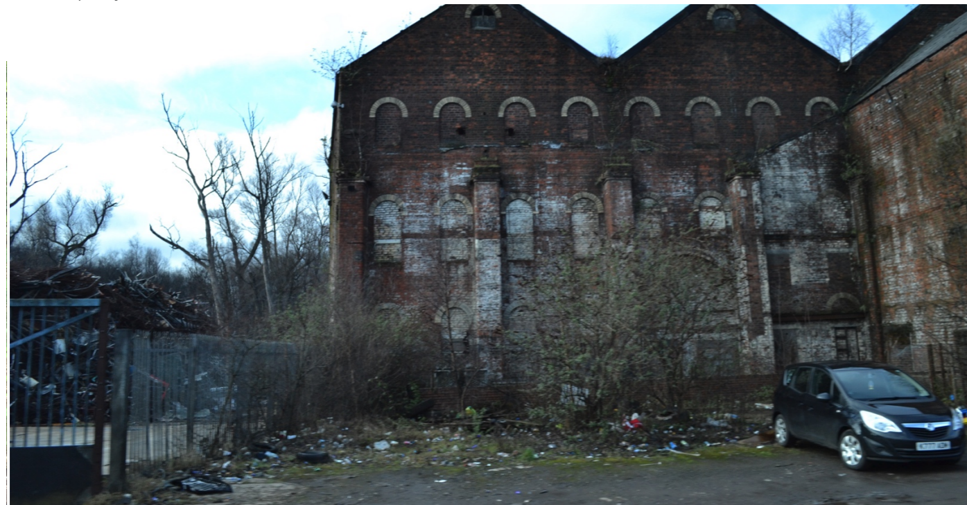
Arched entranceway into building
