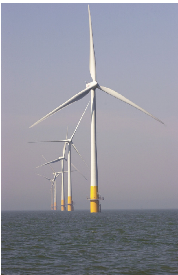
Plate 3.1 3 MW Wind Turbines Installed at the Kentish Flats Offshore Wind Farm (Photographer Chris Laurens)
