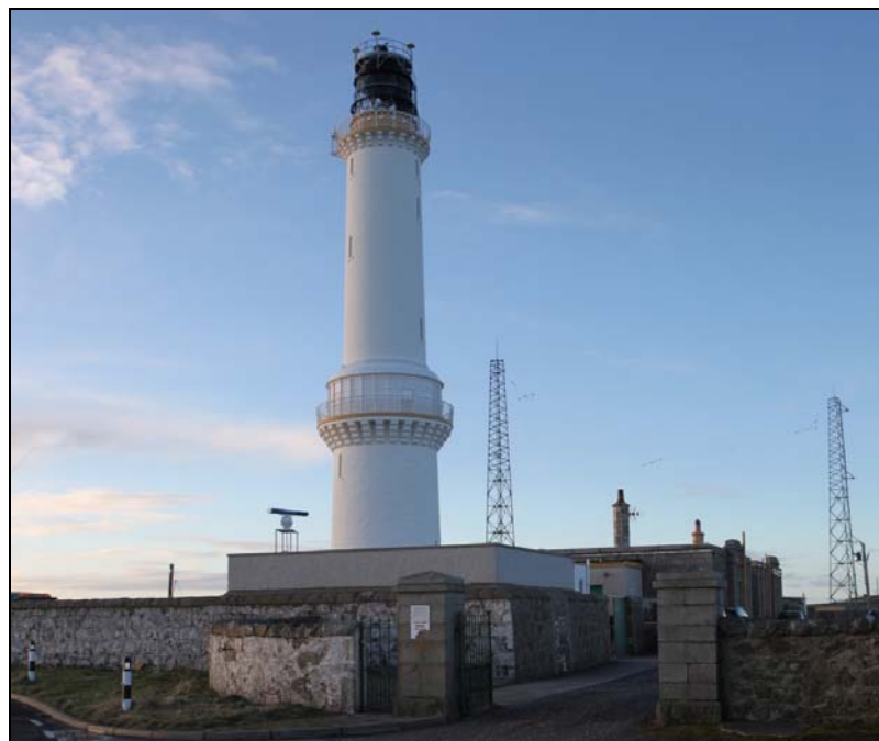
Figure 8.2 Radar Scanner located next to Girdle Ness Lighthouse
