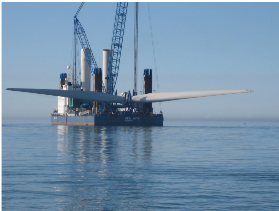
Plate 3.2 Jack Up Installation Barge at Ormonde Offshore Wind Farm
