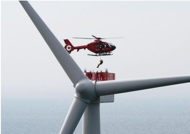
Figure 7.16: A Typical Heli-hoist Platform (Source: SSE)
