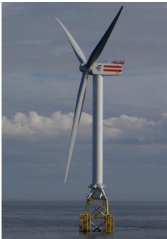
Figure 7.15A: A Representative WTG Access System shown on the Substructure (Source: ICOL)
