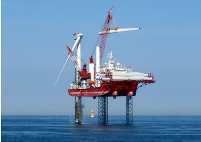
Figure 7.11: Individual Component Installation (Source: Seajacks)
