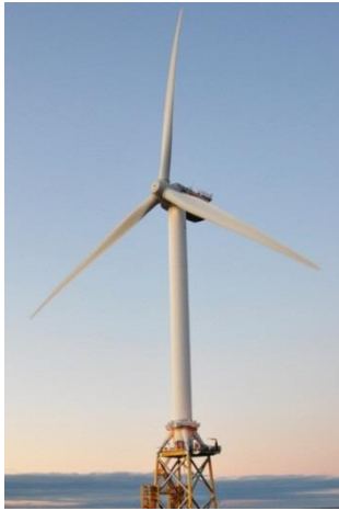
Figure 7.8: A Typical Offshore WTG (Source: ICOL)
