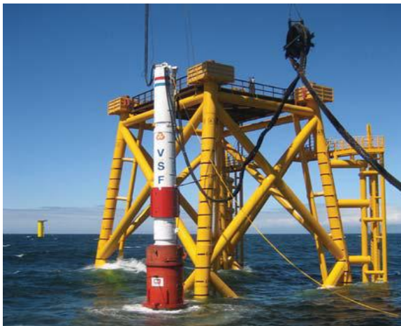
Figure 7.21: A Typical Pile Driving Operation (Source: VSF)
