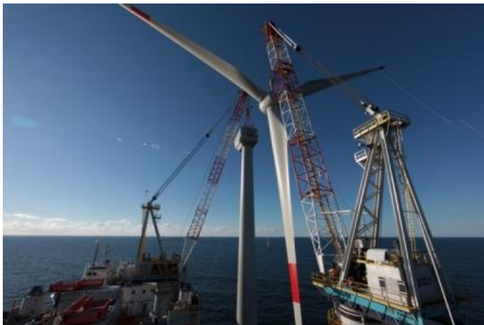
Figure 7.12: Fully Assembled Rotor Installation (Source: AREVA, Alpha Ventus)
