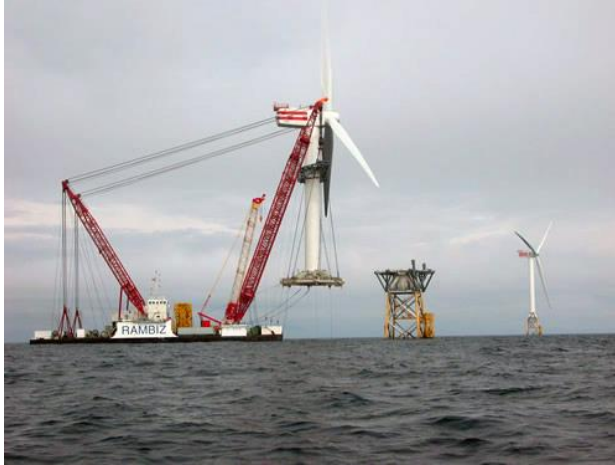
Figure 7.13: Single Lift WTG Installation (Source: SCALDIS)
