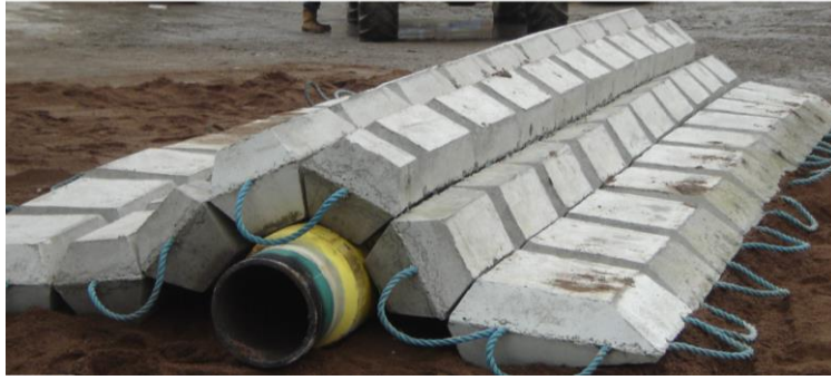
Figure 7.33: Concrete Mattress Laid over a Test Pipe (Source: SPS)
