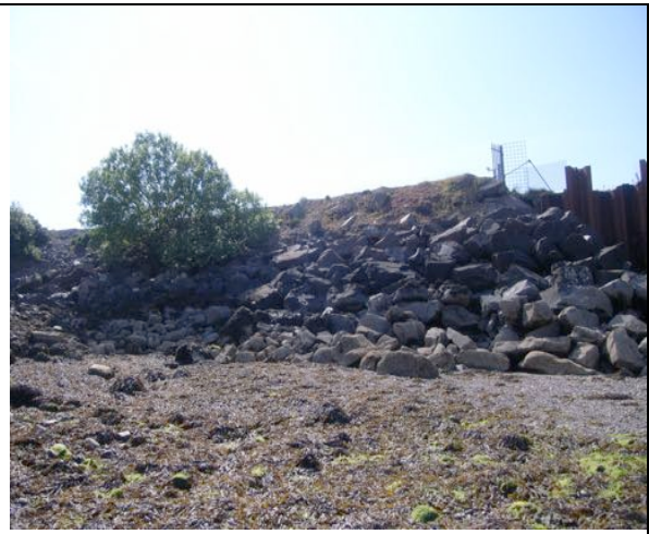
Looking at the east side of the pier at Intertidal area where new slipway would impinge. Cavities in the rip-rap by the willow tree are suitable for otter shelters. June 2016, photo 78.
