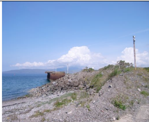
H1.2 & H3 Looking northwards at the west side of the pier at the rip-rap placed to protect the pier – security fence visible at inner end of pier; June 2016, photo 12.
