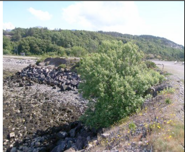
Looking west from pier track at part of the inter-tidal area with cobbles, where a new slipway would be built. June 2016, photo 71.
