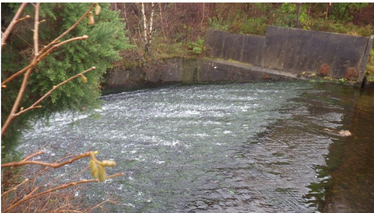
Figure A-3 Allt Anavig reservoir overflow weir crest and spillway
