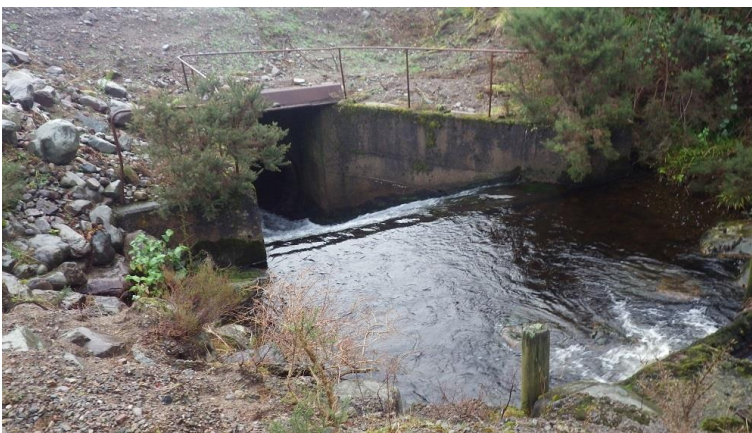
Figure A-5 Allt Anavig culvert inlet
