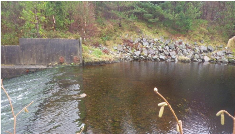
Figure A-2 Allt Anavig reservoir overflow weir crest
