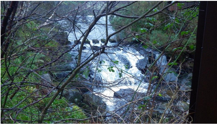
Figure A-4 Allt Anavig reservoir overflow weir crest and spillway
