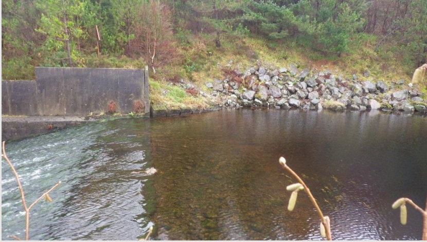
Figure A1.4 Alt Anavig –spillway at the reservoir outlet, showing accumulations of finer sediments (gravel and silt) retained behind concrete crest, concrete wing walls and boulder revetments approximately 1.8-2.0m above water level.
