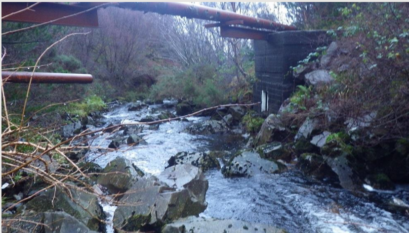
Figure A1.2 Alt Anavig downstream of A87, showing large boulders exposed within plane channel and additional revetment at pipe crossing point on face of left bank.
