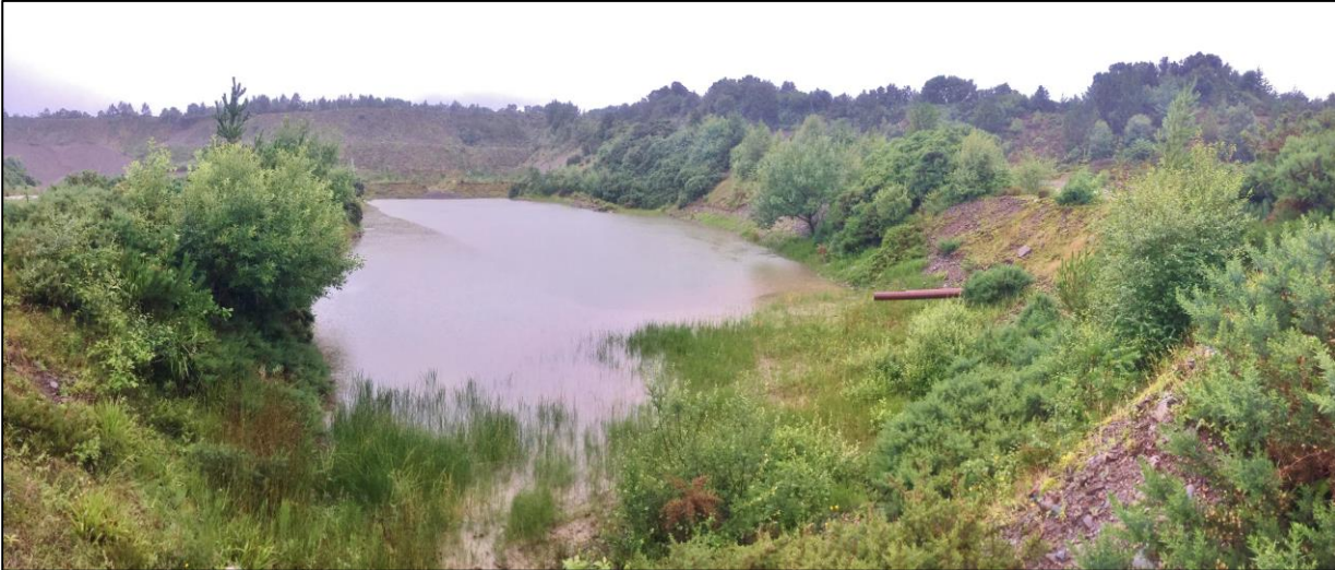
Photograph 11.1 : Settlement pond showing drainage pipe and marginal vegetation.
