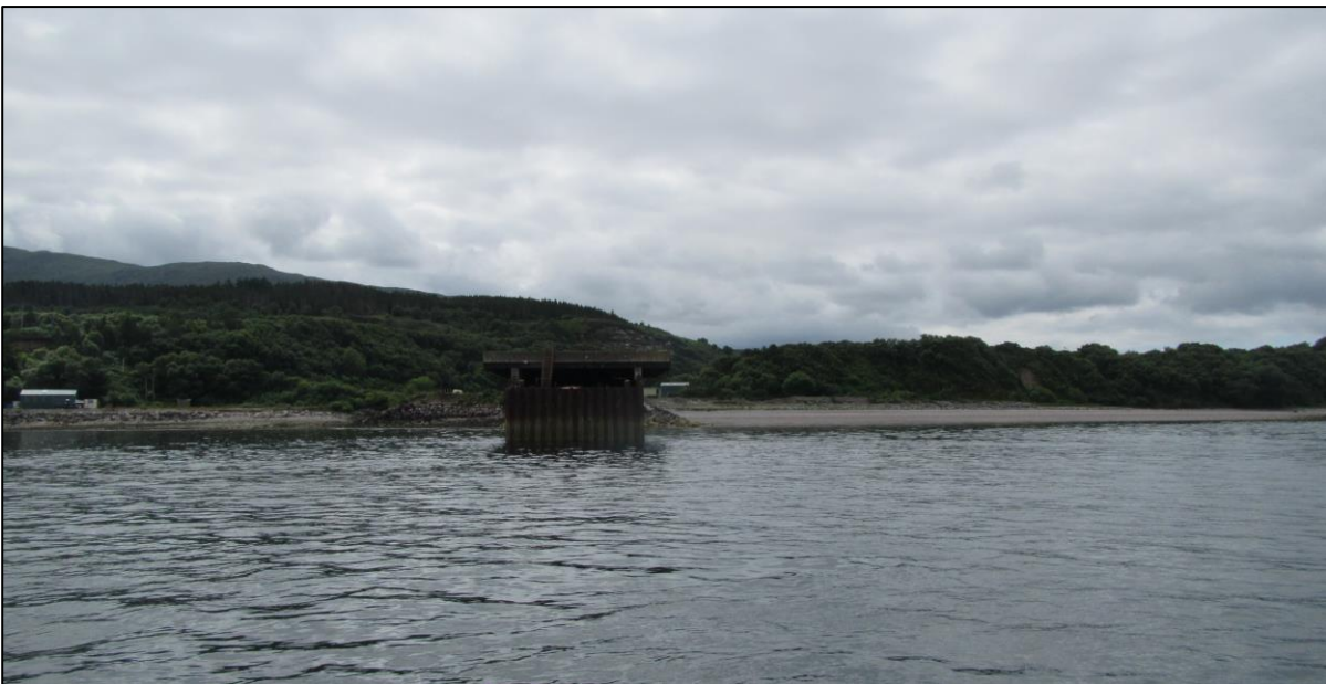
Figure 19.3 : View of shoreline looking south towards the existing pier. Rock armouring can be seen at southern base of pier with a continuation of rock armour along the upper shore to the east of the pier.
