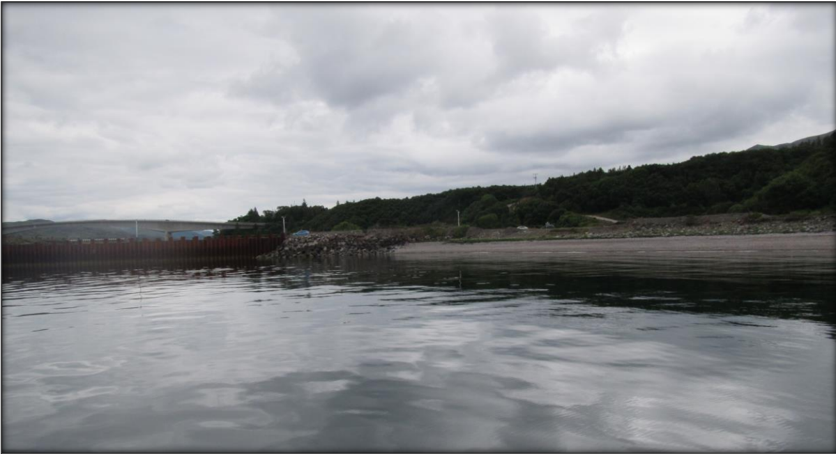
Figure 19.2 : View of shoreline looking east towards the existing pier. Rock armouring can be seen at southern base of pier.
