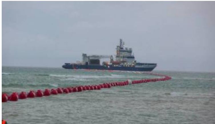
Figure 8.6 Cable floated / pulled ashore from a DP Cable Lay Vessel
