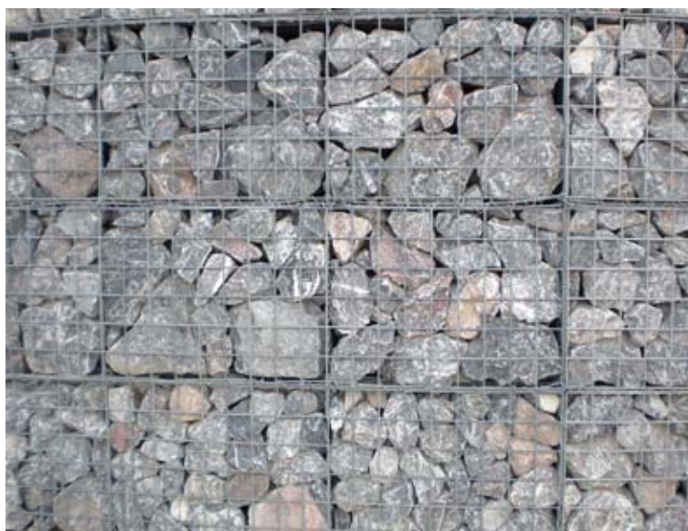
Figure 8.5 Typical Gabion Basket / Reno Mattress
