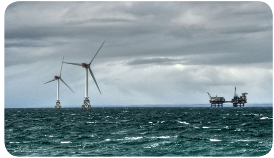
Above: Beatrice Demonstration Turbines and Beatrice Oil Field
