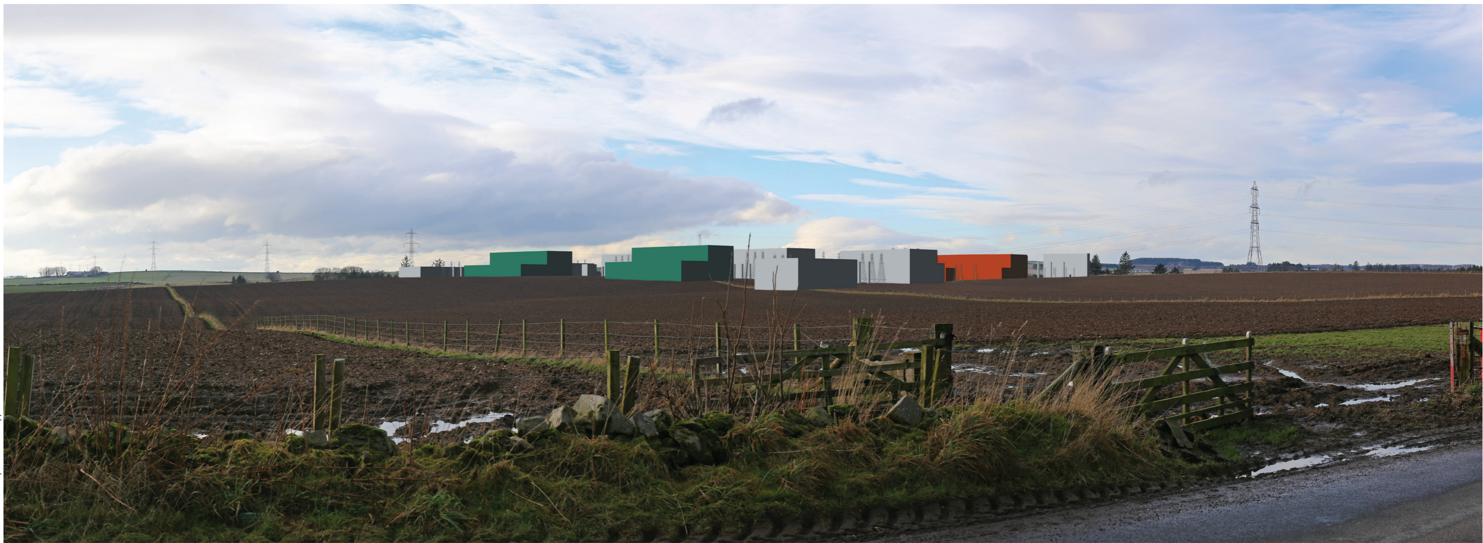
Photomontage view showing the development envelopes for the proposed onshore substations. Camera: Canon EOS 5D Mark II Focal Length: 50mm Horizontal Field of View: 72 degrees Camera Height: 2m Date: 04/02/14 Time: 15:08
