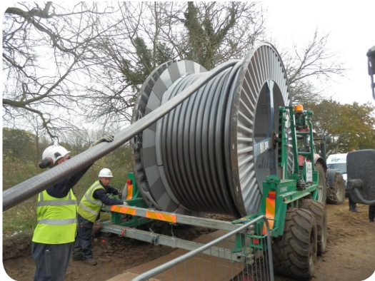
Left Top: cable duct installation, Left Bottom: cable pull (cable drum)
