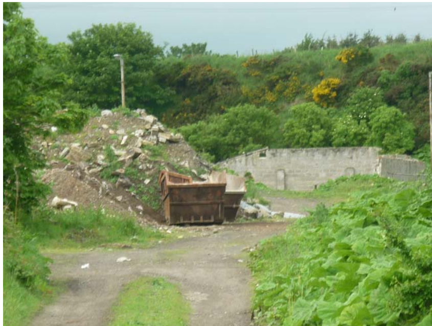
Photograph 5: Demolition rubble at Inverboyndie
