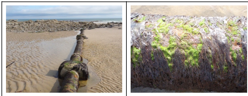
Plate 4.1 Existing pipe present to the west of the proposed cable route
