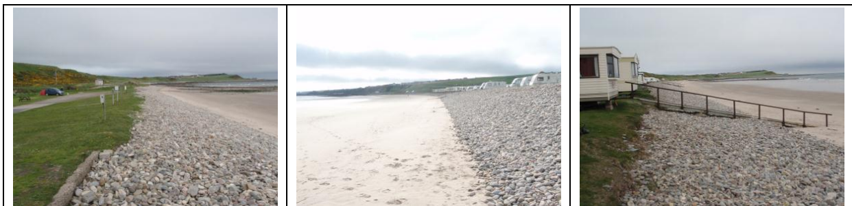
Plate 4.2 Gravel/pebble rock armour on the eastern side of the survey area
