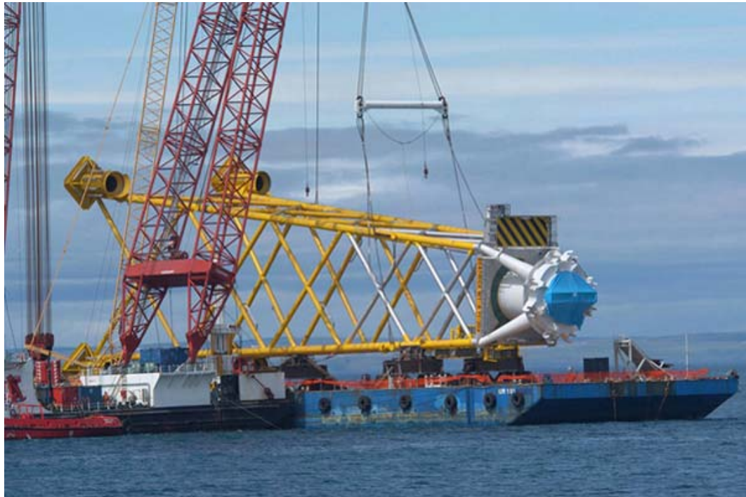
Figure 1-3: Photo of the jacket foundation used at the Beatrice OWF
