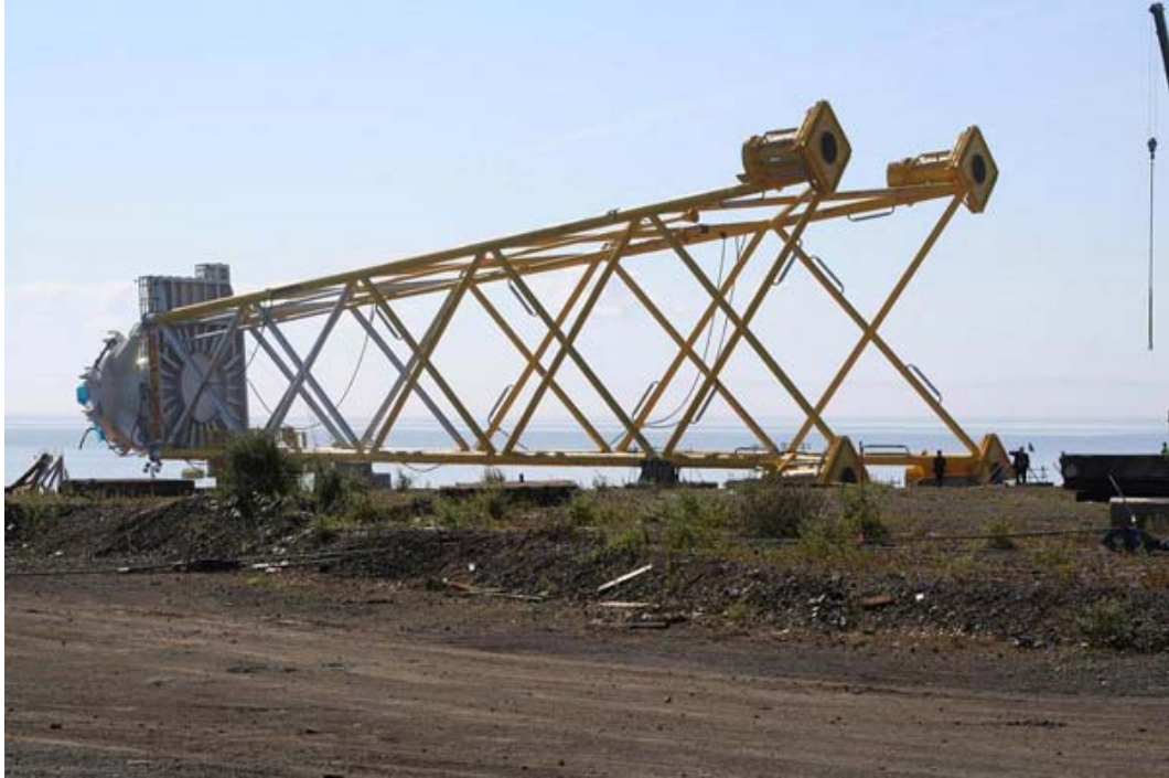
Figure G- 13 : Photographs of the jacket structure used the Beatrice OWF site
