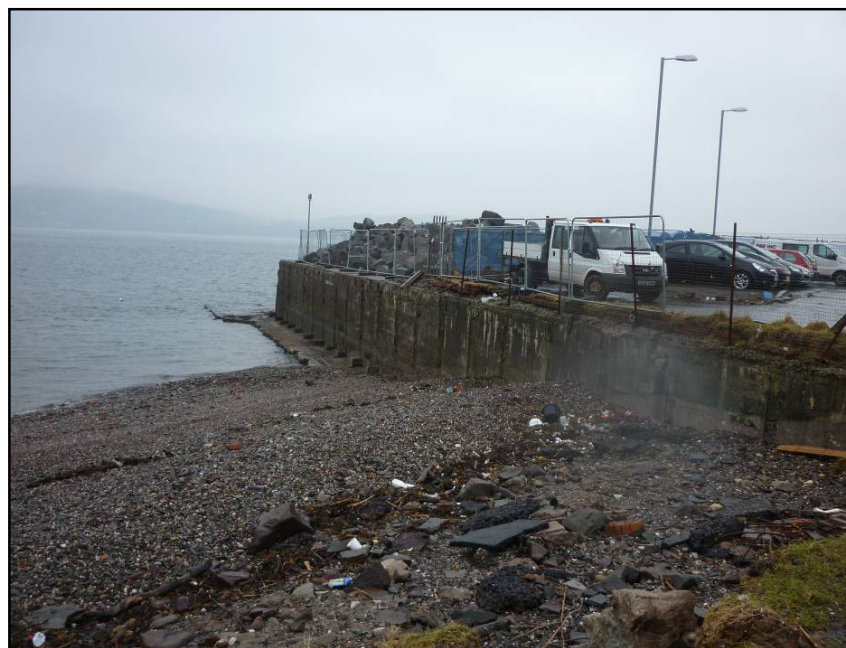
Photograph 2.3 – Pierhead to North of Station Car Park
