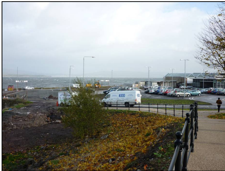
Photograph 2.1 – Station Car Park
