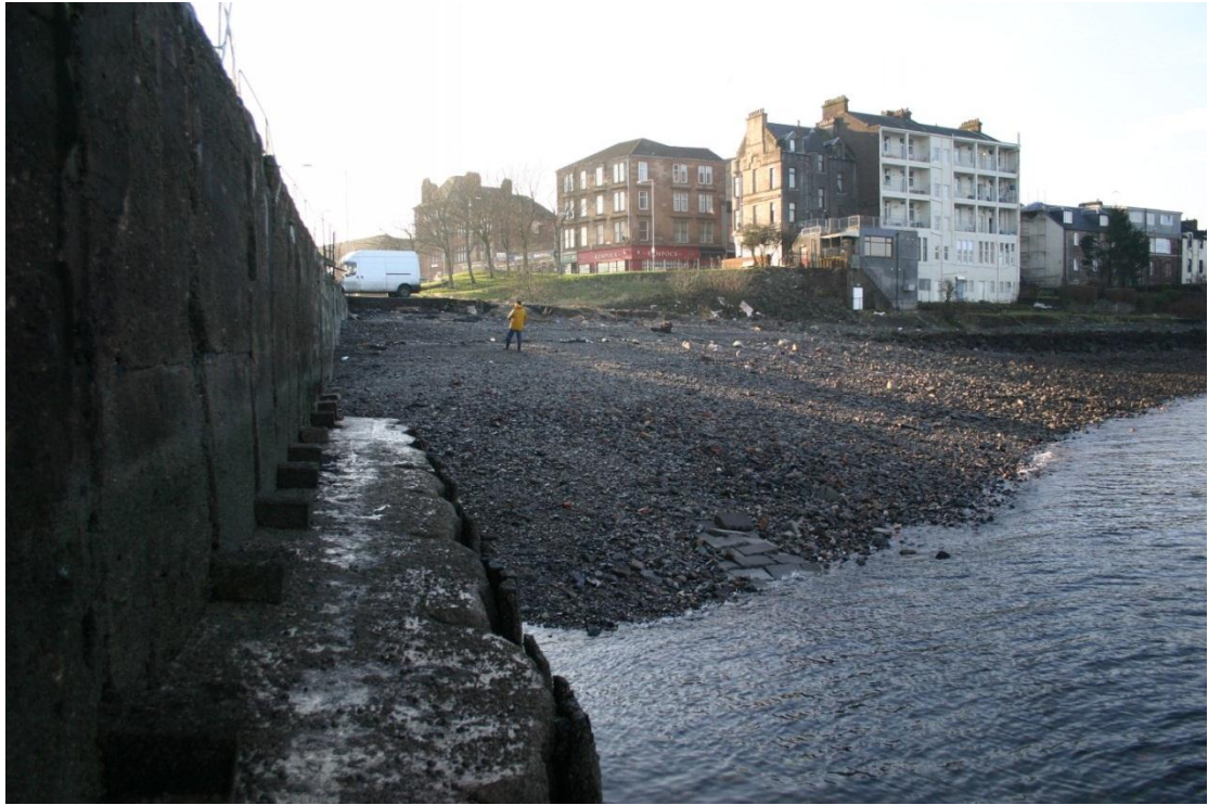
Plate 9: Looking South from north-western extent of Survey Area
