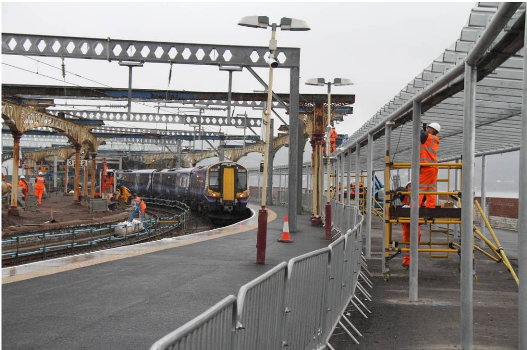
Gourock Station ferry terminal walkway refurbishment
