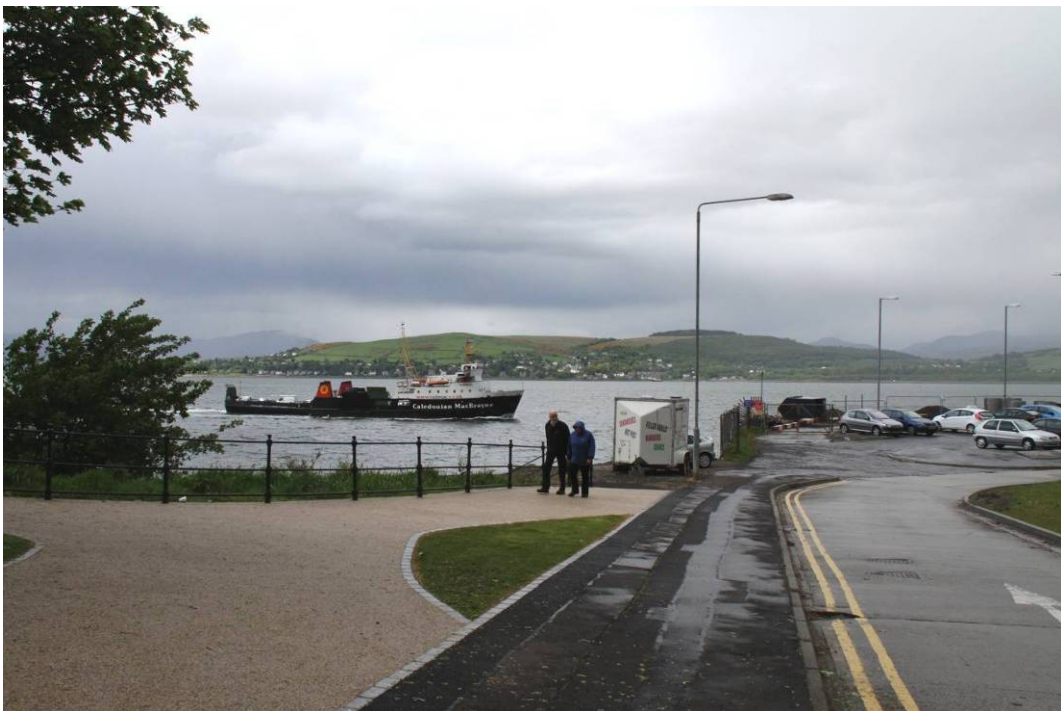
Pedestrian footway and footpath improvements west of Station Car Park
