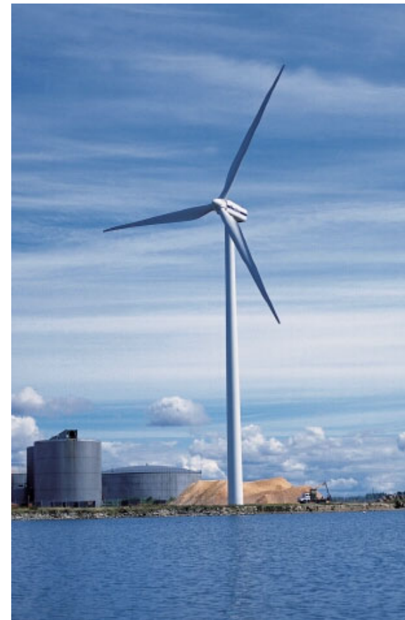
Figure 4.6.1 2 MW V80 Turbine (Courtesy of Vestas wind Systems A/S)
