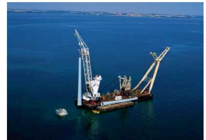
Figure 4.17.3 Floating crane vessel. (Courtesy Vestas Wind Systems A/S)
