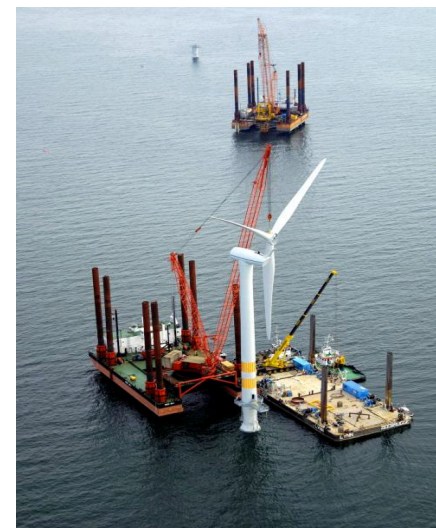
Figure 4.17.2 Jack-up barge (Courtesy Seacore Ltd)
