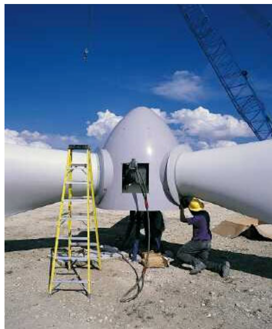
Figure 4.16.1 Assembly of Rotors Onshore
