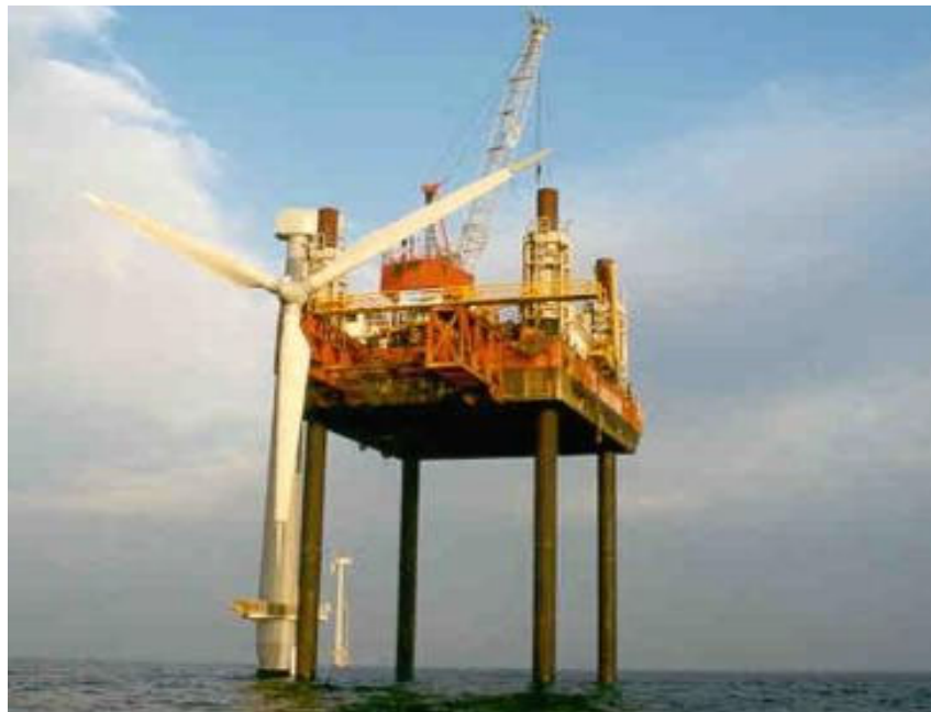
Figure 4.17.5 Installation of Rotor (Courtesy Seacore Ltd)
