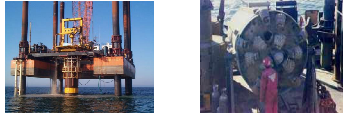
Figure 4.17.4 Drilling for installation of monopile foundation (Courtesy SeacoreLtd)
