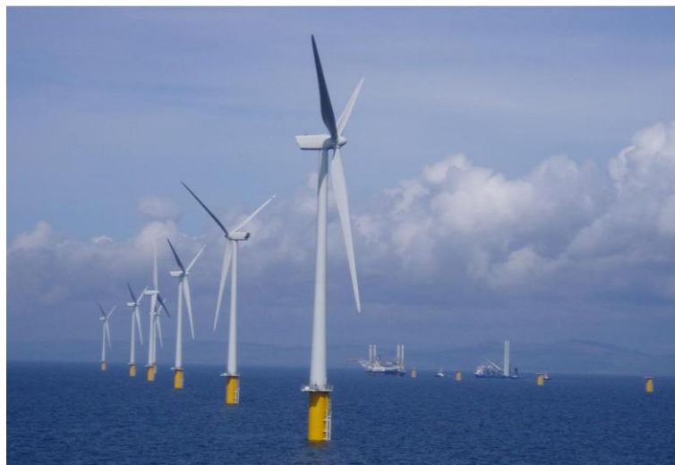
Figure 1.1c: Photograph of Robin Rigg Offshore Wind Farm during the construction phase.
