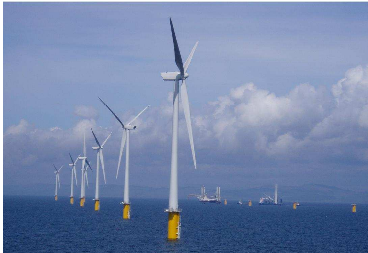
Figure 1.3: Photograph of Robin Rigg Offshore Wind Farm.
