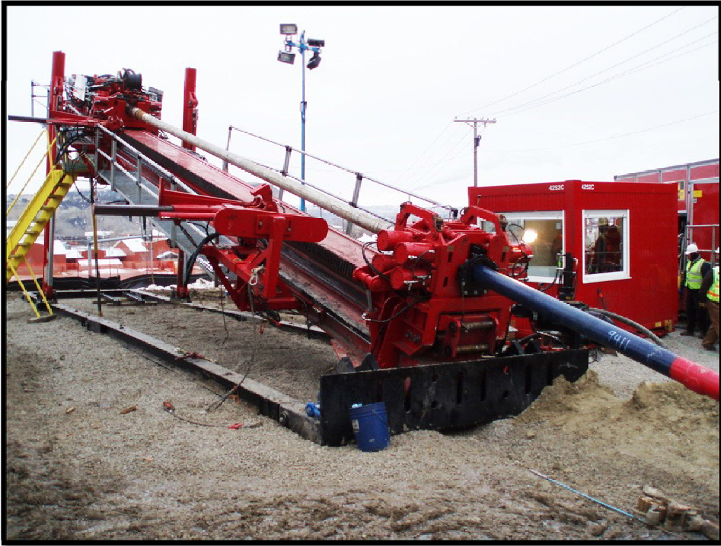
Figure 3: Horizontal Directional Drill Rig.
