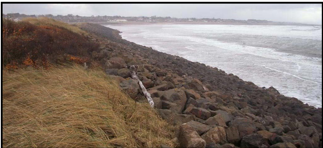
Figure 17 - Sea defences at Carnoustie at the proposed landfall location
