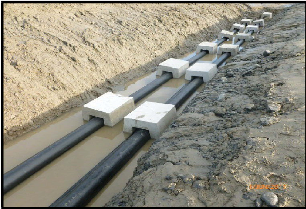
Figure 4: Open Cut Trench Cable Installation
