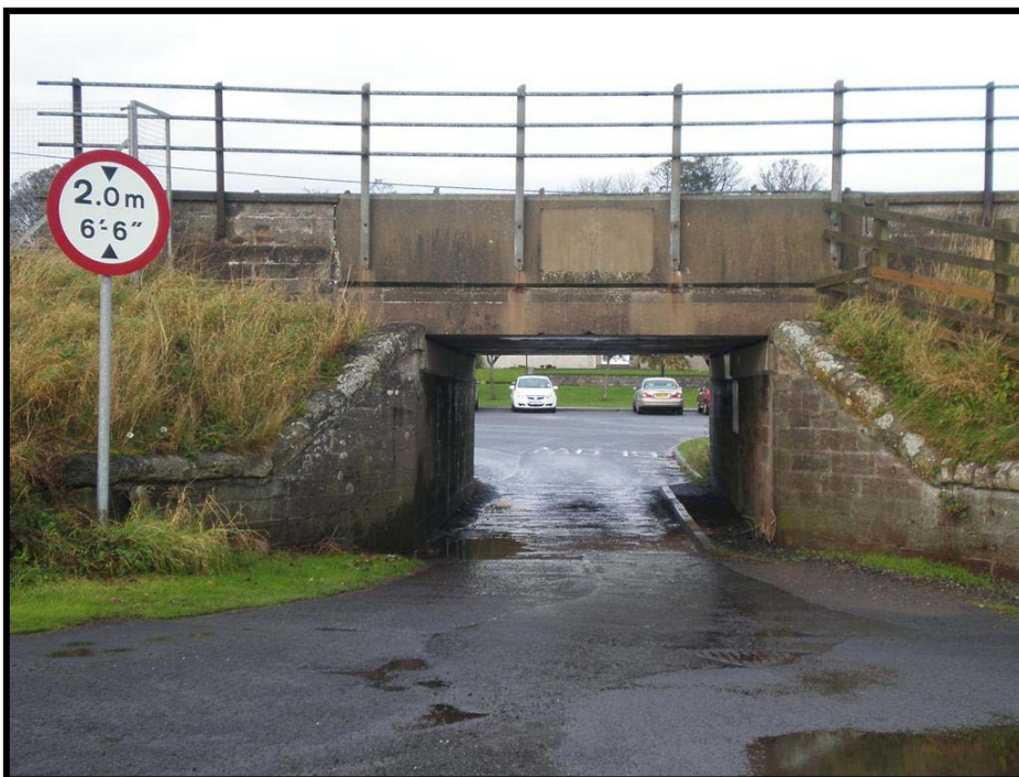
Figure 13. East Haven Construction Beach Access.
