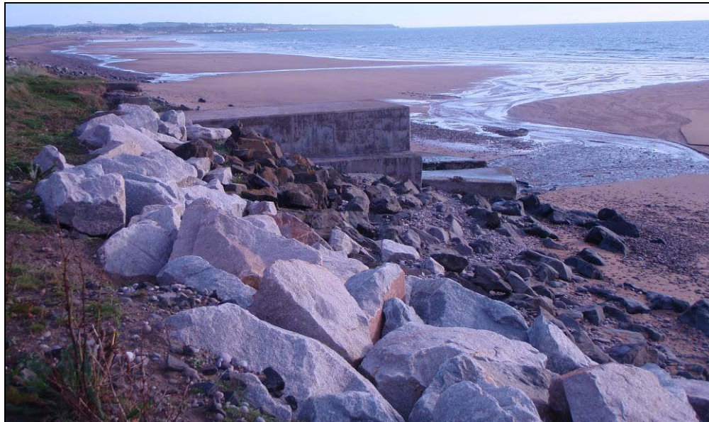
Plate 4.20 Rock revetment within the ECR corridor fronting the low-lying land behind
