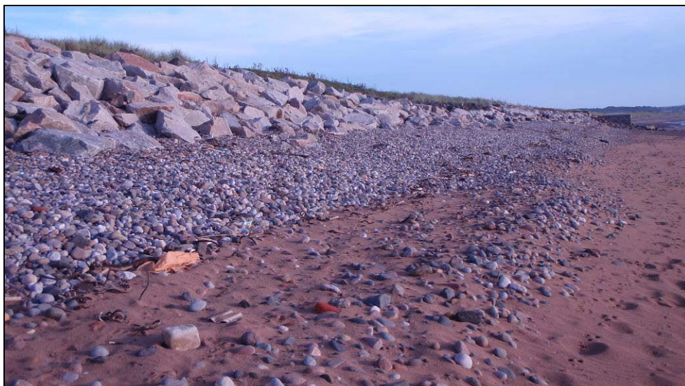
Plate 4.19 Rock revetment within the ECR corridor fronting the low-lying land behind
