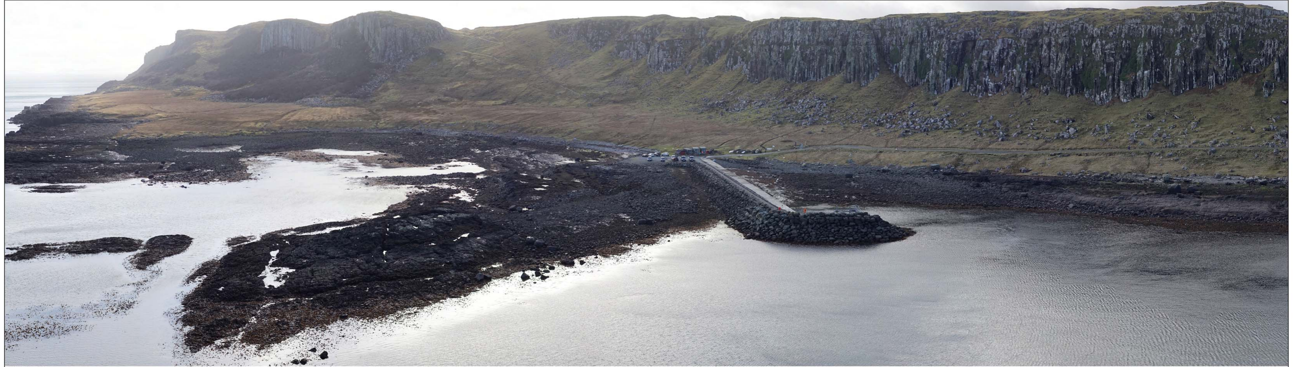
Viewpoint 1A - Existing Photograph
