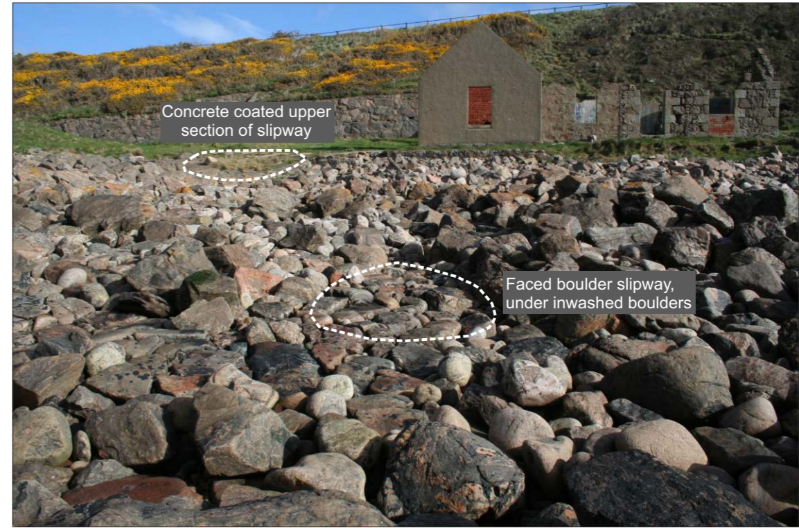
B. Slipway and roofless building
