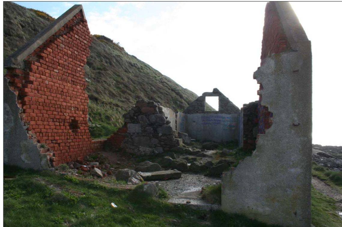
C. Roofless building
