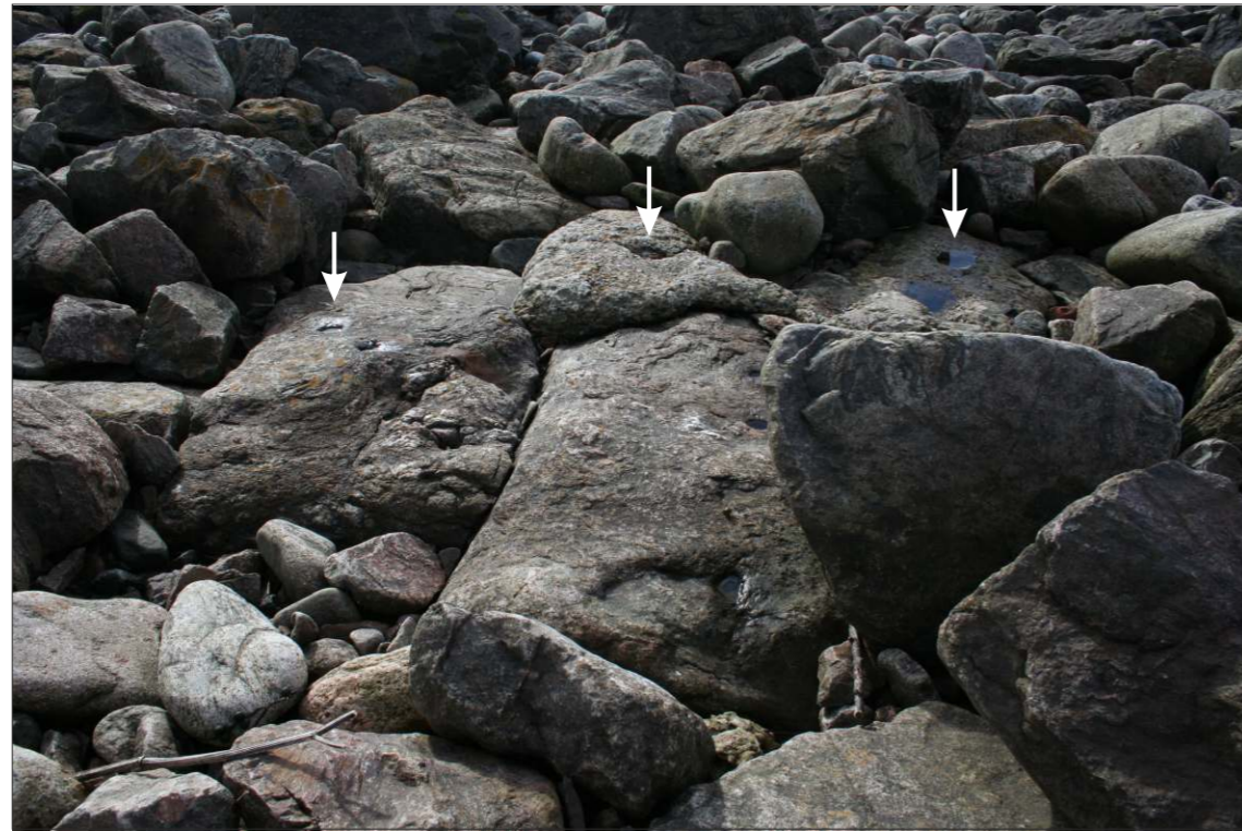
A. Slipway (fastenings highlighted by arrows)
