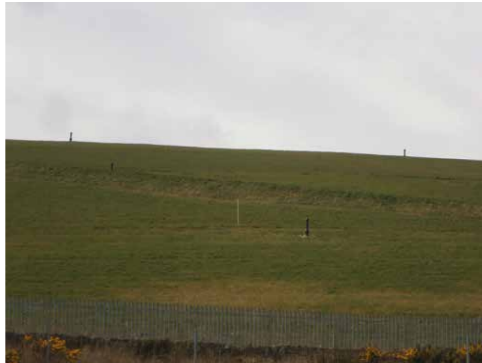
Plate 5: Gas vent pipes on former landfill
