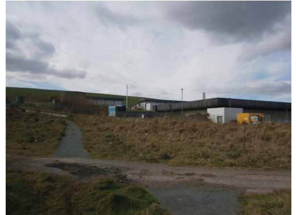
Plate 3: Waste Water Treatment works to the west
