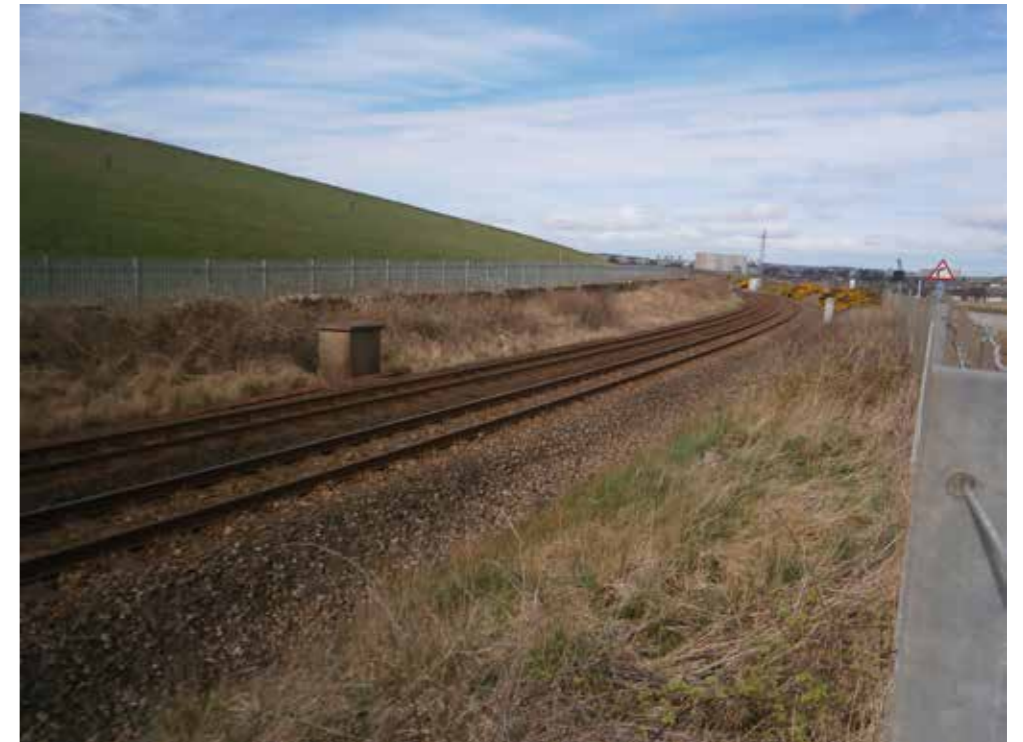
Plate 6: Railway line adjacent to the site boundary
