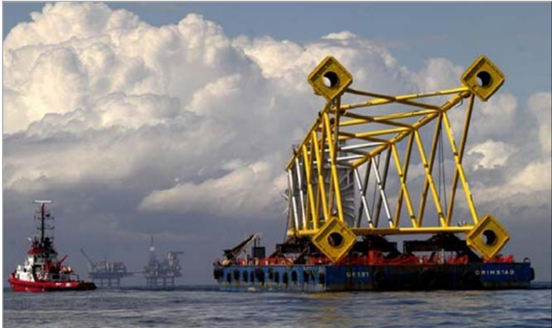
Plate 7.7 Tug Towing Lattice Jacket Substructure on Pontoon Barge
