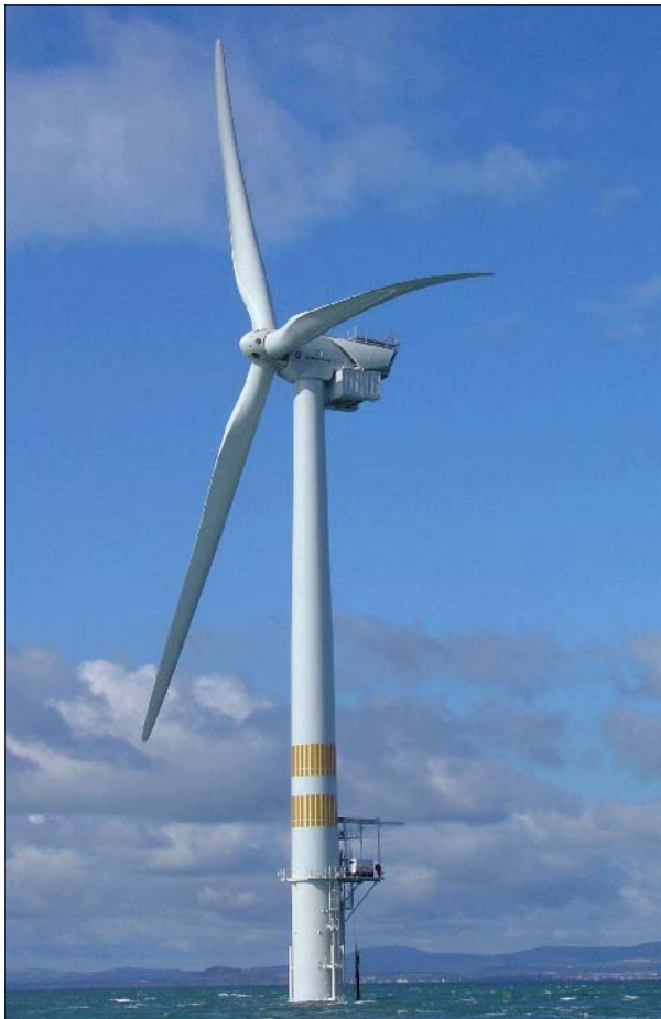
Plate 7.1 Typical Offshore Turbine
