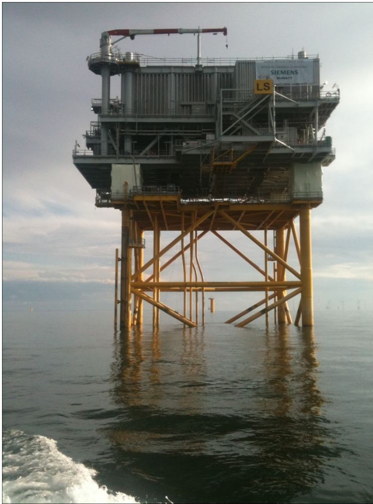
Plate 7.4 Indicative Offshore Substation Platform (OSP)
