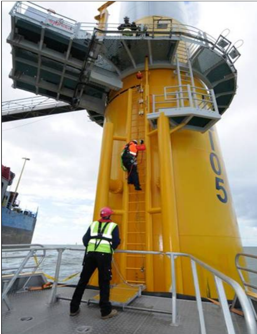
Plate 7.2 Typical Turbine Boat Landing and Access Facility
