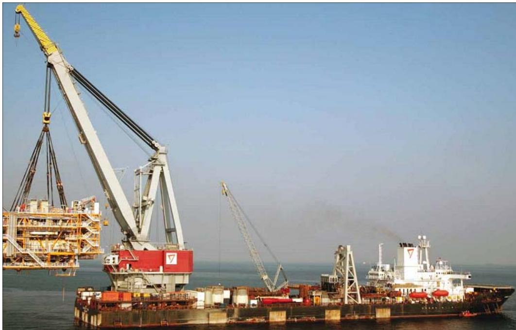
Plate 7.3 Single Lift Activity undertaken by Heavy Lift Vessel
