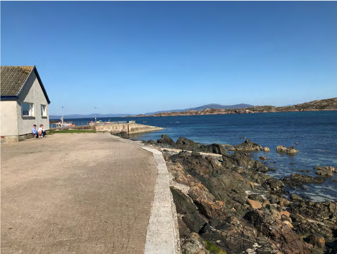
Plate 1: Existing jetty seen from the south
