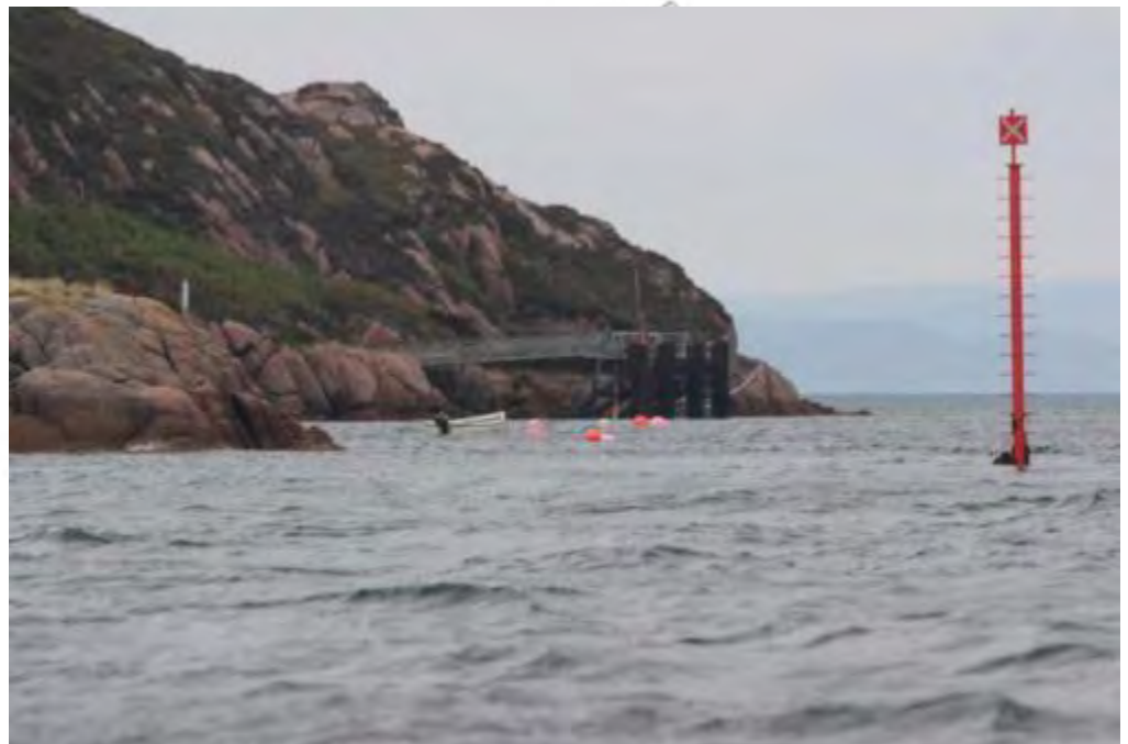
■ Figure 3-3 Berthing at Bull Hole
