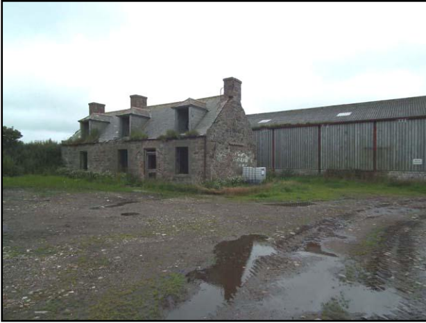
Photo 22. Old building, potentially highly suitable habitat for roosting bats (NK030491, TNE15)
