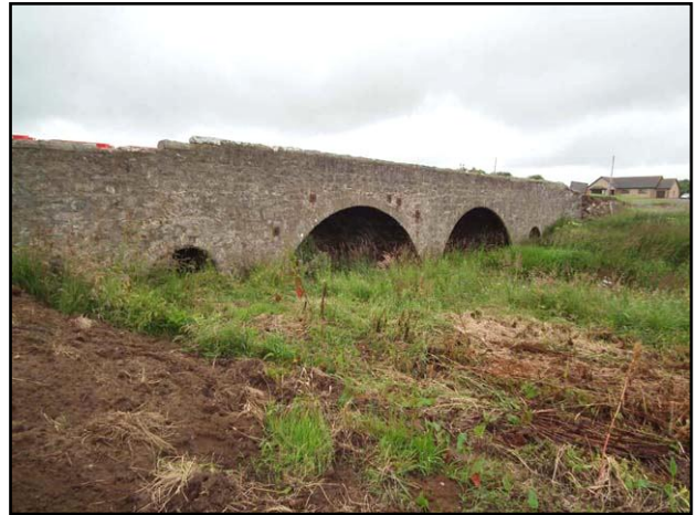
Photo 25. Bridge, potentially highly suitable habitat for roosting bats (NK041492, TNE10B)
