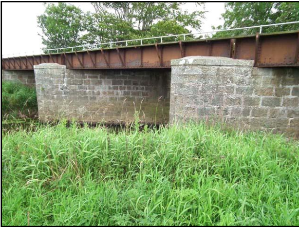
Photo 24. Bridge, potentially highly suitable habitat for roosting bats (NK052481, TNE5)
