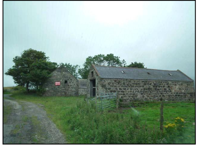
Photo 23. Old building, potentially highly suitable habitat for roosting bats (NK014517, TNE28C)
