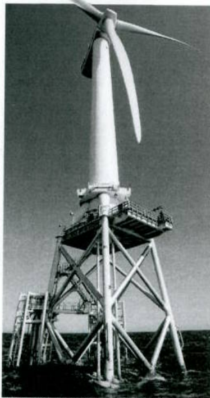
The underground power cable will transport electricity from wind turbines in the outer Moray Firth to Inverboyndie and on to two new sub-stations near New Deer.
