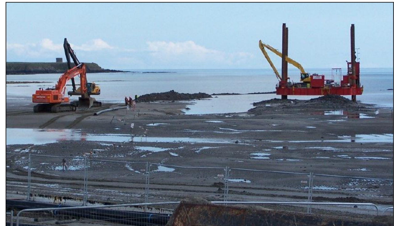
Figure 5.33: Beach excavations – tracked excavators and barge mounted excavators (Source ETA Ltd)
