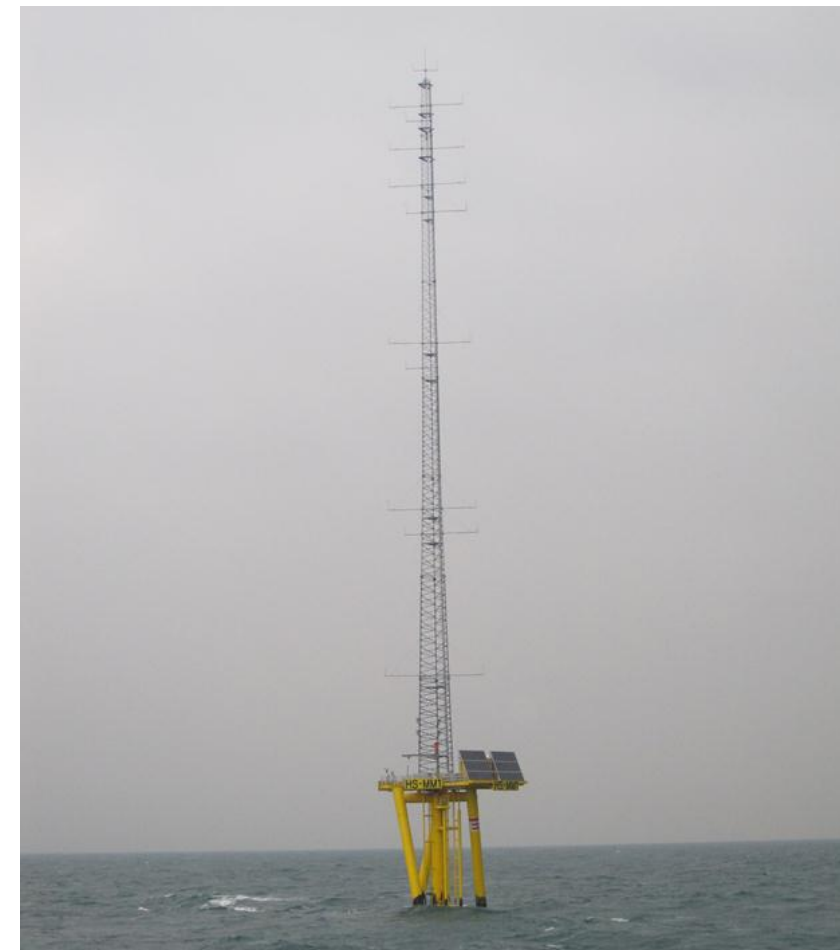
Figure 5.2: Example met mast at Hornsea offshore wind farm (Source: SMart Wind)
