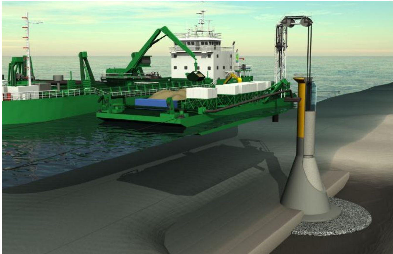
Figure 5.11: Schematic of vessel used for filling gravity base foundation (Source: DEME Group)
