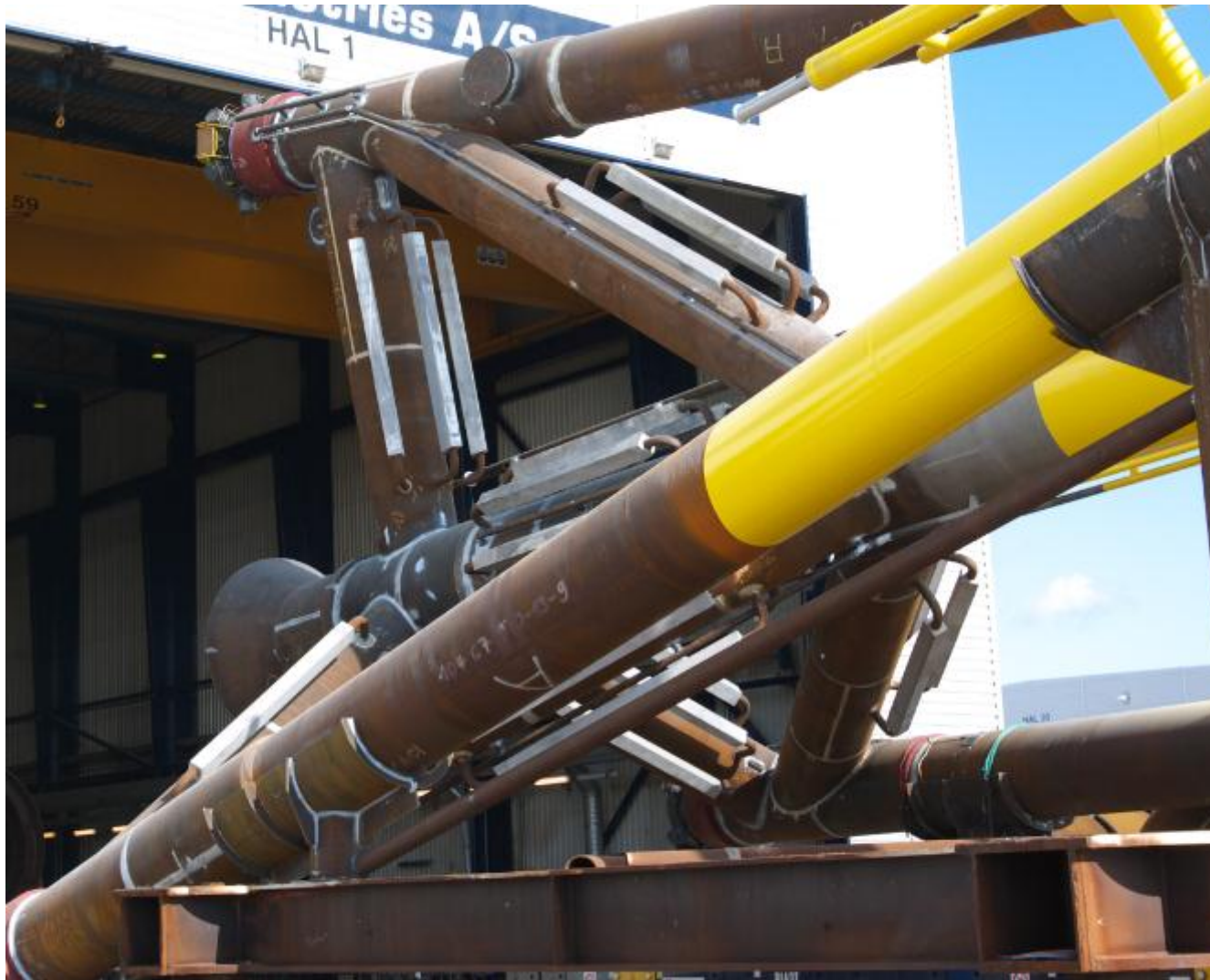
Figure 5.14: Anodes affixed to jacket members (source: Keystone)
