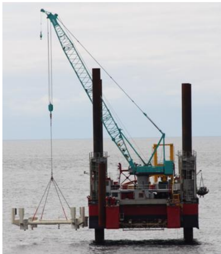
Figure 5.16: Jack-up barge installing seabed template (source: Fugro Seacore)
