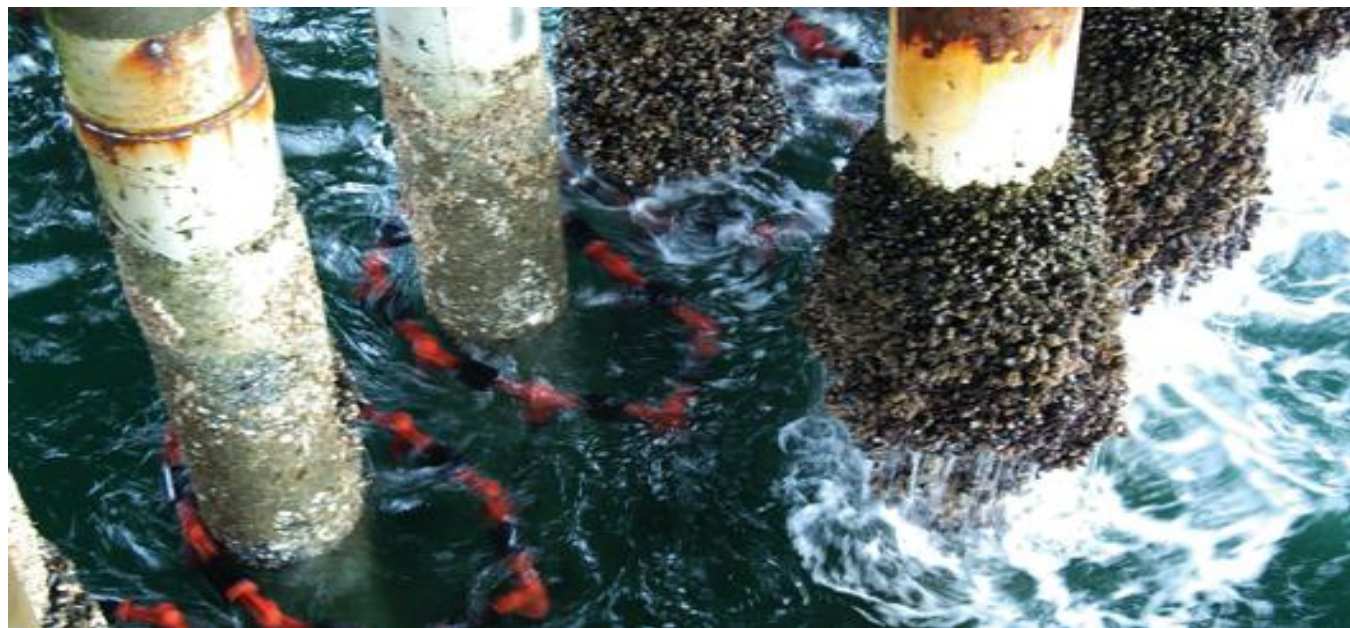
Figure 5.34: Marine growth prevention solutions (Source: FoundOcean Ltd)
