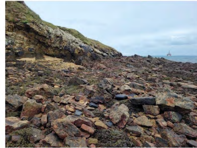
Plate 3d. Scapa Deep Water Quay intertidal survey Transect 3 (SB_3), view south from the upper shore.
