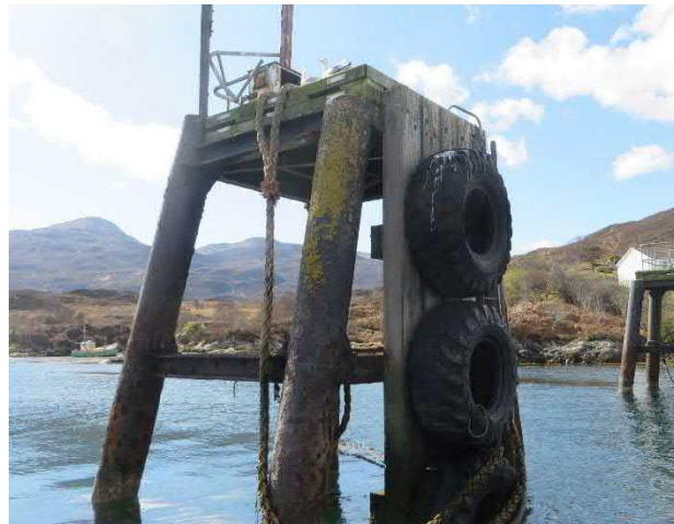
Figure 2.2: Outer berthing dolphin (with nav light)
