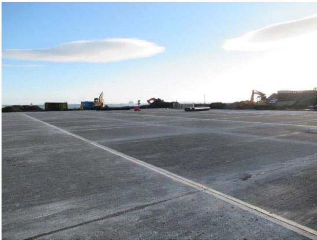
New extended quayside decommissioning area
