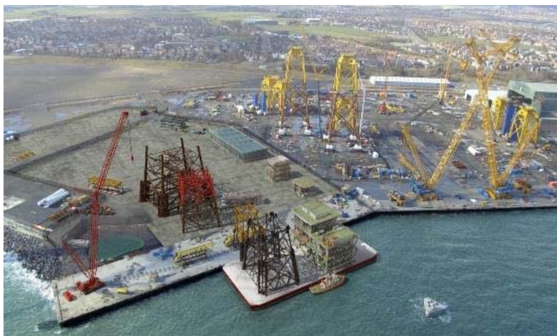
Fife Energy Park CGI of CessCon Decom Facility (New decom slab complete and buildings consented behind existing quays. Existing BiFAB yard to east)
