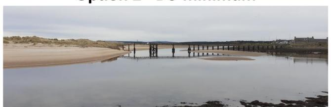
Under the do-minimum scenario the superstructure would be limited to the footprint and self-weight of the existing structure. The existing footbridge is approximately 1.2 metres wide between parapets and 120 metres long.
